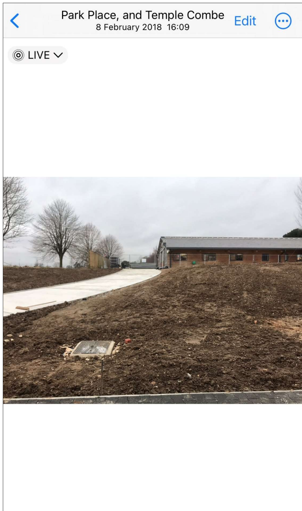
Photo. 1 – Shows construction of the concrete link way between Park Place stable buildings (shown) and the polo stable block.
