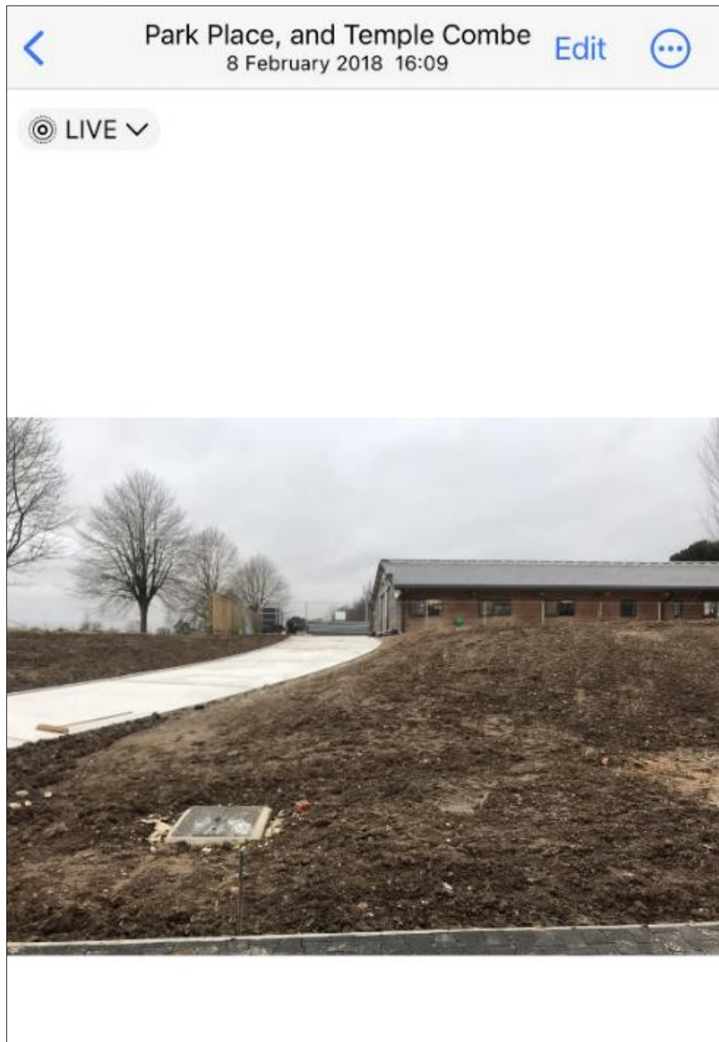
Fig. 7 – Smartphone photo taken by A Price showing construction of the concrete link way
