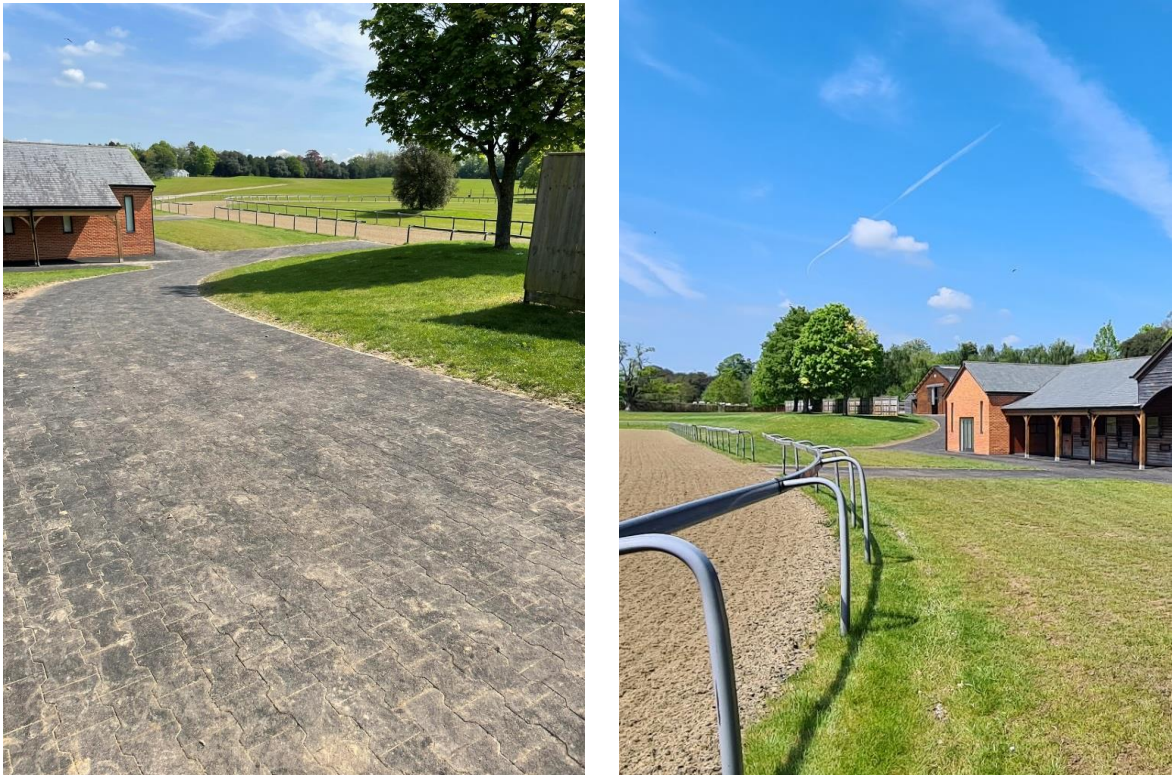
Fig. 4 – The rubberised matting link way (May 2024)
