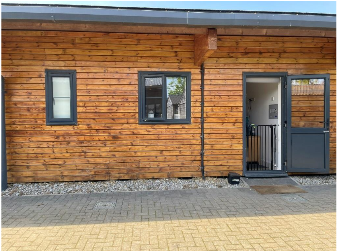
Fig. 1 - Front door and main entrance point into accommodation
