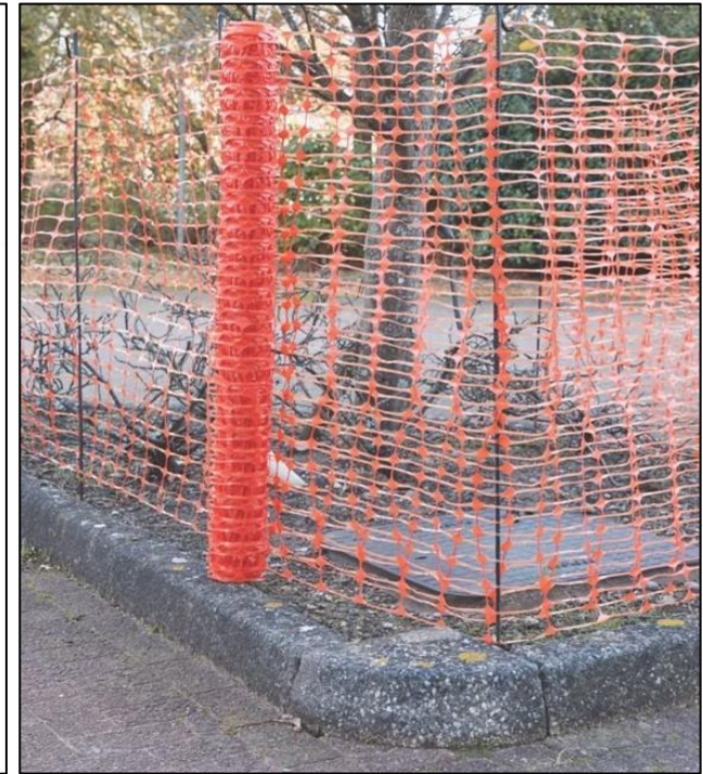
Image 3: Showing orange netlon fencing supporting by road pins.
