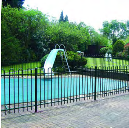
LDS: Black anti-trap bow top railing with high contrast colour gates Dimensions: 1200mm height above ground Example shown: Jacksons fencing tubular bowtop railing R13: Landform and ornamental planting have been used to provide boundaries to the play space
