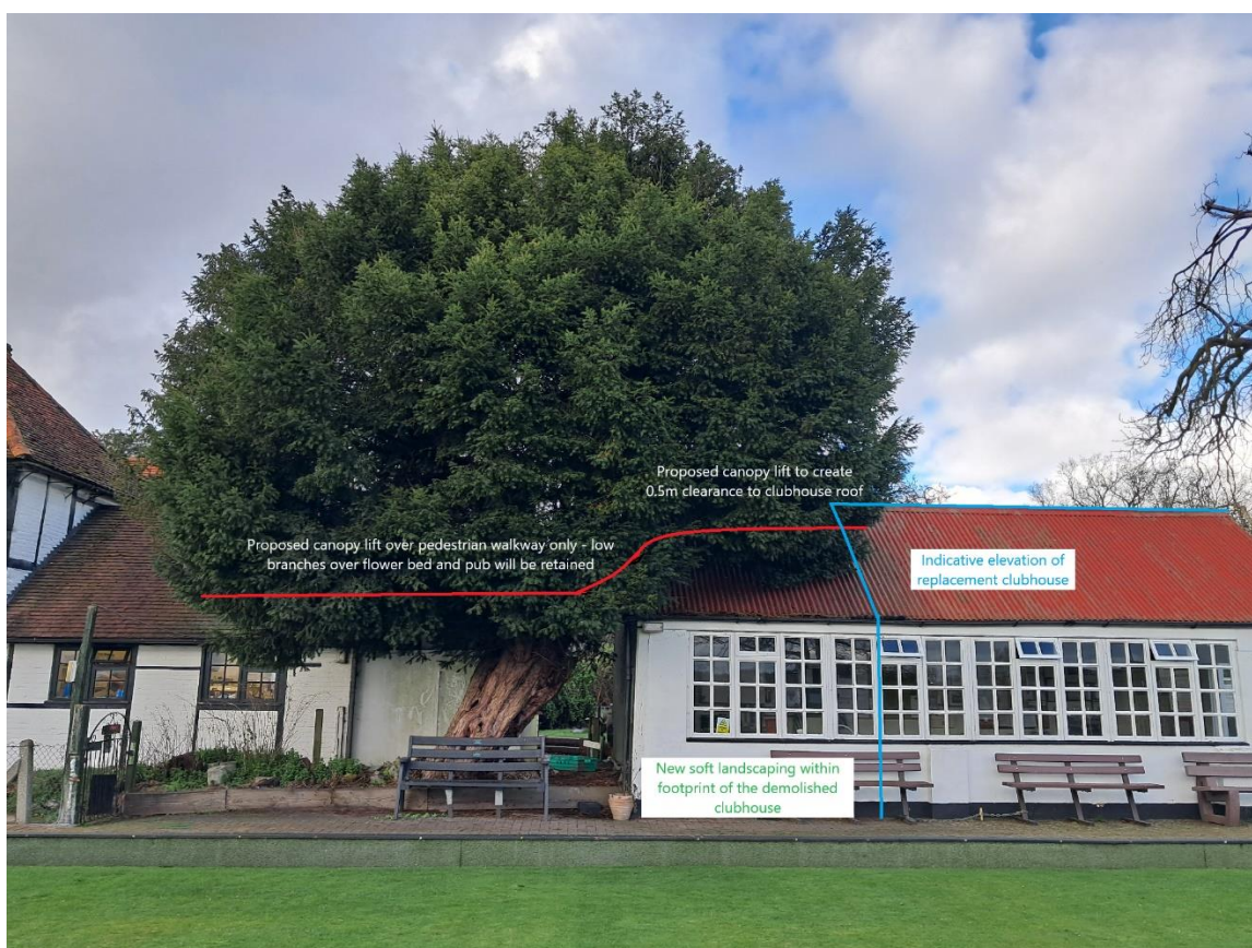
Photo 2 – Indicative height of proposed canopy lift as viewed from the south
