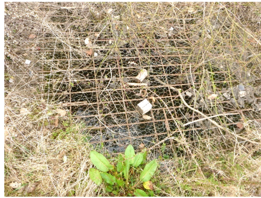
Photograph 13. Drain at the base of the bank.
