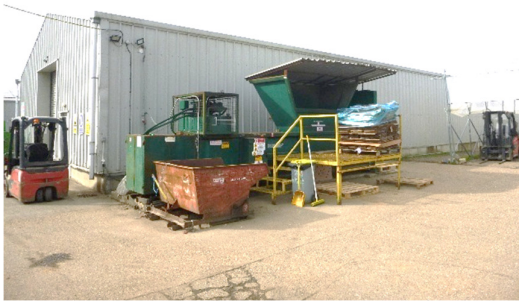
Photograph 3. Warehouse towards the north of the site.
