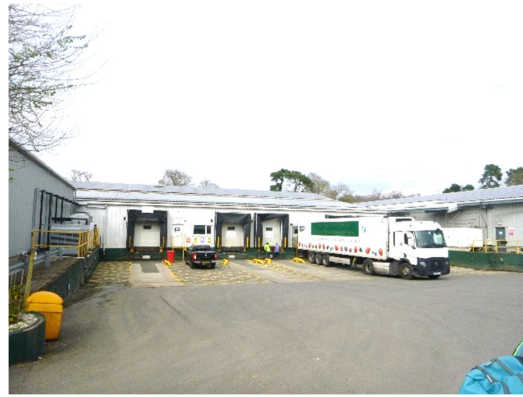
Photograph 4. Warehouse towards the north of the site.
