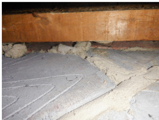
Photograph 15. Gaps along gable filled with mortar.
