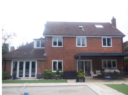
Photograph 2. Rear of property viewed from south.
