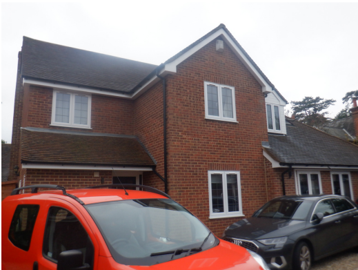
Photograph 1. Front of property viewed from north.
