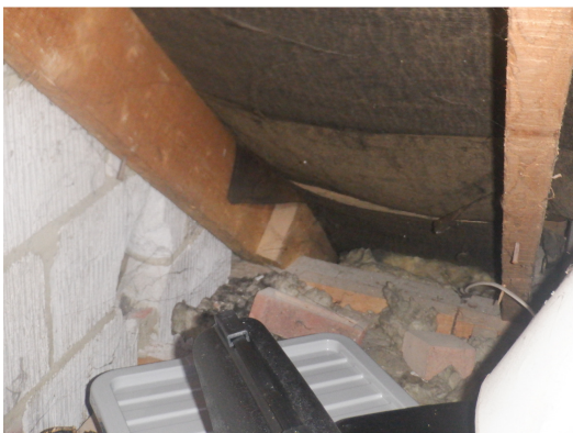
Photograph 14. Eaves filled with fibreglass insulation.
