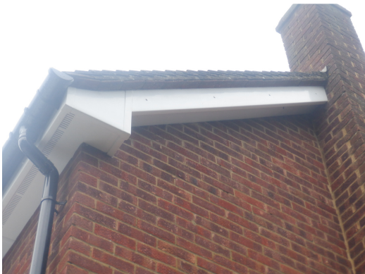
Photograph 9. uPVC soffit sealed to the brickwork gable (eastern elevation)
