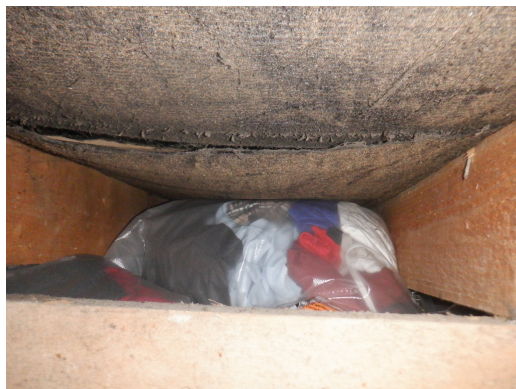
Photograph 13. Overlapping sections of bitumen felt.
