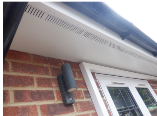
Photograph 10. uPVC soffit sealed to the brickwork (front elevation).
