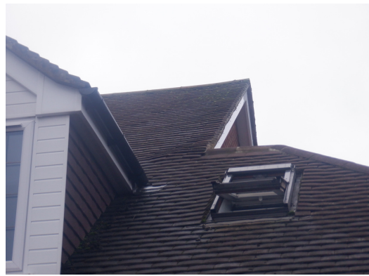
Photograph 4. Raised verge roof tiles (front elevation).
