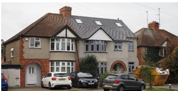
Fig 1: Frontage as built
