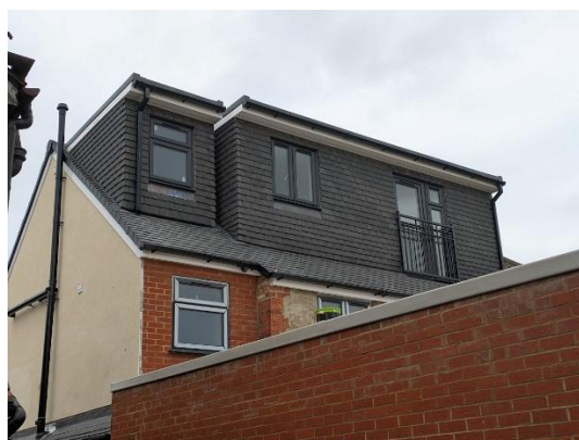
Fig 4: Two Obtrusive Dormers As-Built Note stack pipe
