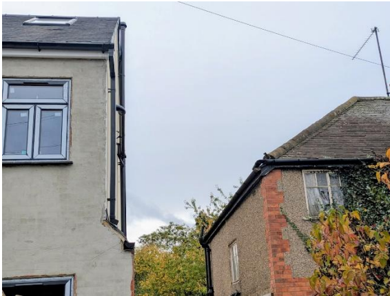
Fig 5: Dominance and overbearing of the side extension with respect to 26
