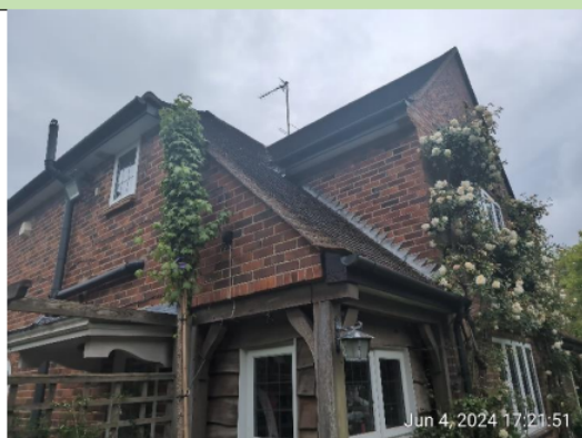
Figure 5: B1 south-eastern corner
