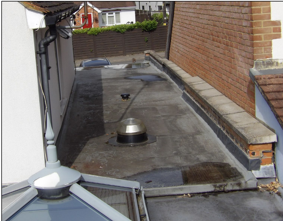
Figure 12. Well fitted PVC membrane on garage. 44 Bearwood Road, Wokingham. 15.07.25
