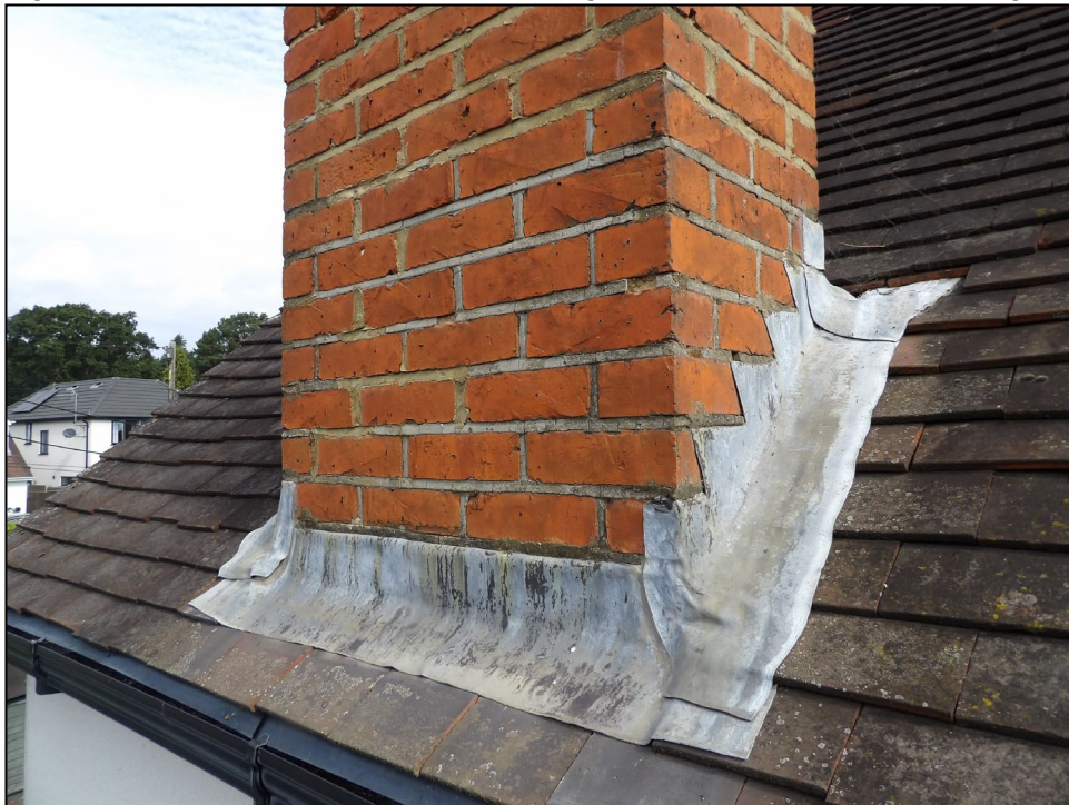
Figure 6. Example of sealed lead flashing. 44 Bearwood Road, Wokingham. 15.07.25
