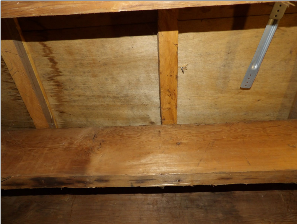
Figure 15. Interior view of garage roof. 44 Bearwood Road, Wokingham. 15.07.25
