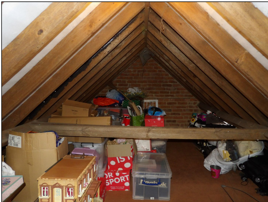
Figure 13. Example loft space and membrane lining. 44 Bearwood Road, Wokingham. 15.07.25
