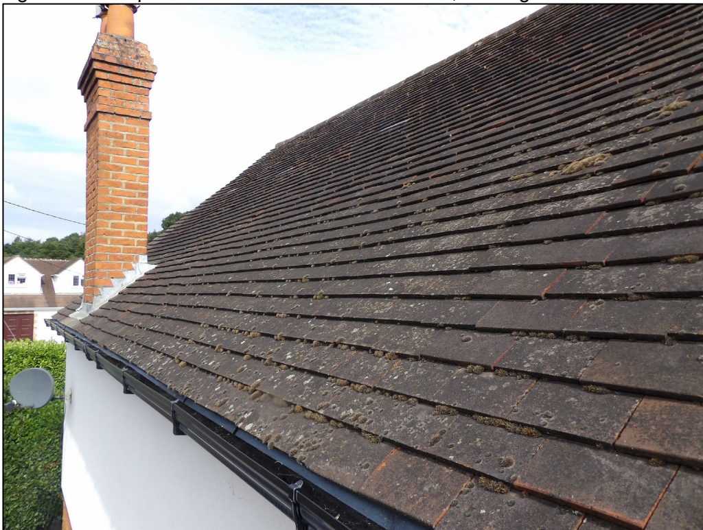
Figure 4. Example of roof tiles. 44 Bearwood Road, Wokingham. 15.07.25
