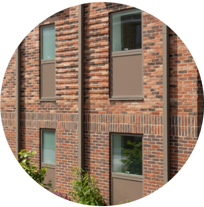
Brick Detailing: Soldier Coursing and Corduroy detailing provide a defined plinth at street level Burlington Close Housing, Kendall Kingscott Architects
