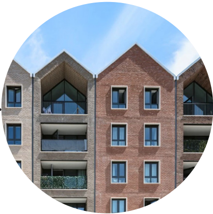
Gables provide frontage and focus for key elevations and views Egham Gateway, Runnymede AHMM Architects
