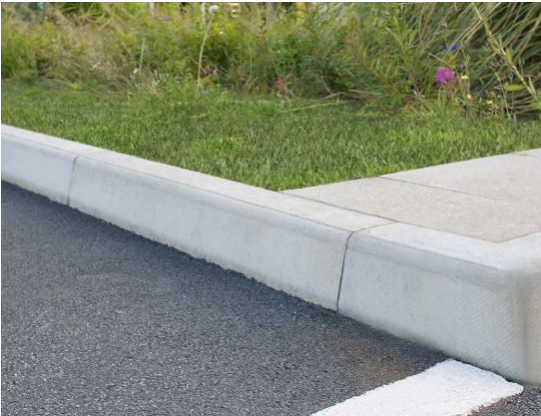
Standard Concrete Kerb (Half battered)
