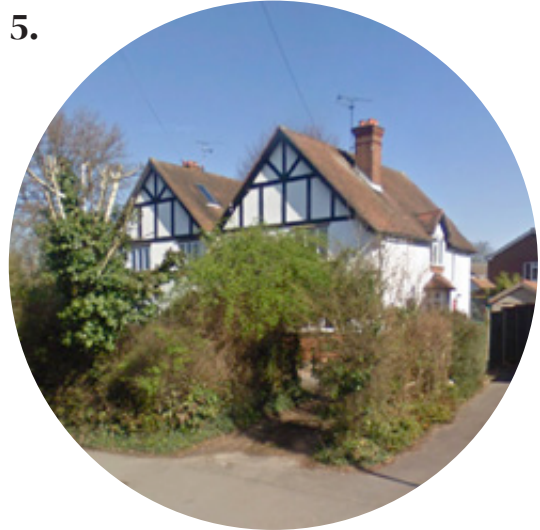
Wellington Road houses adjacent to the site
