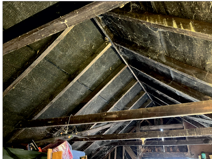
Photograph 4: Showing the inside of the outbuilding, which was heavily cobwebbed throughout.
