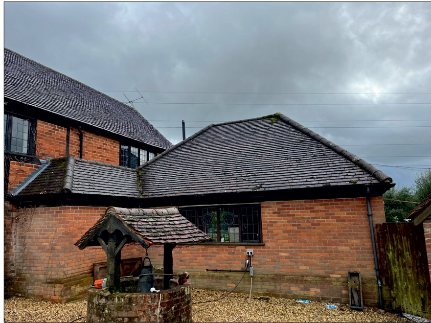
Photograph 1: Showing the front of the single-storey extension.
