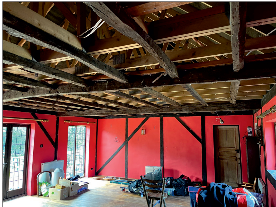
Photograph 3: Showing the internal structure of the single-storey extension.
