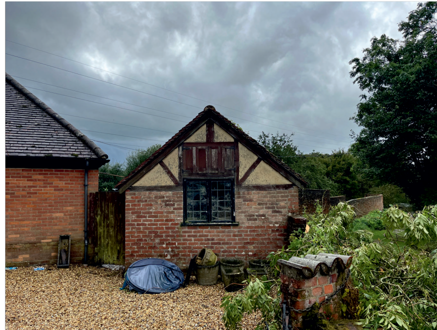
Photograph 2: Showing the front of the outbuilding.
