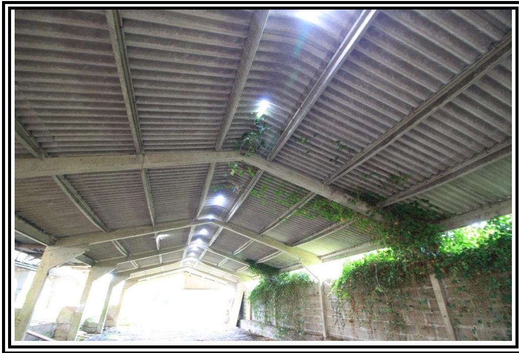
Photo 9: Building CD –internal view Part D
