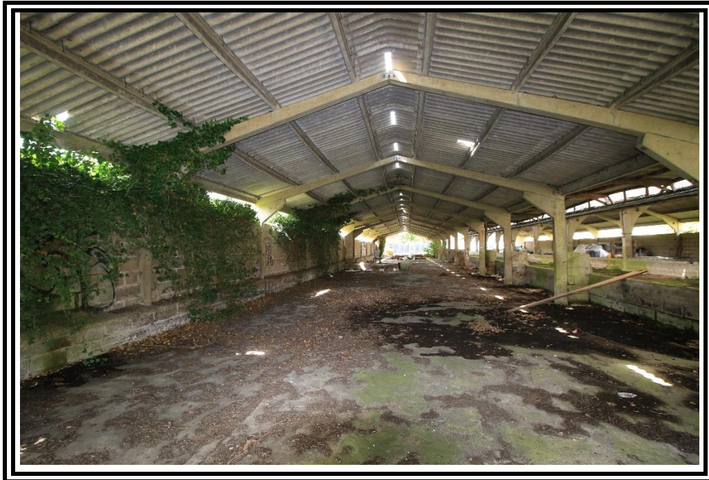
Photo 8: Building CD –internal view Part D
