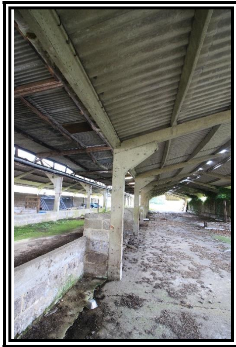
Photo 11: Building CD –internal view
