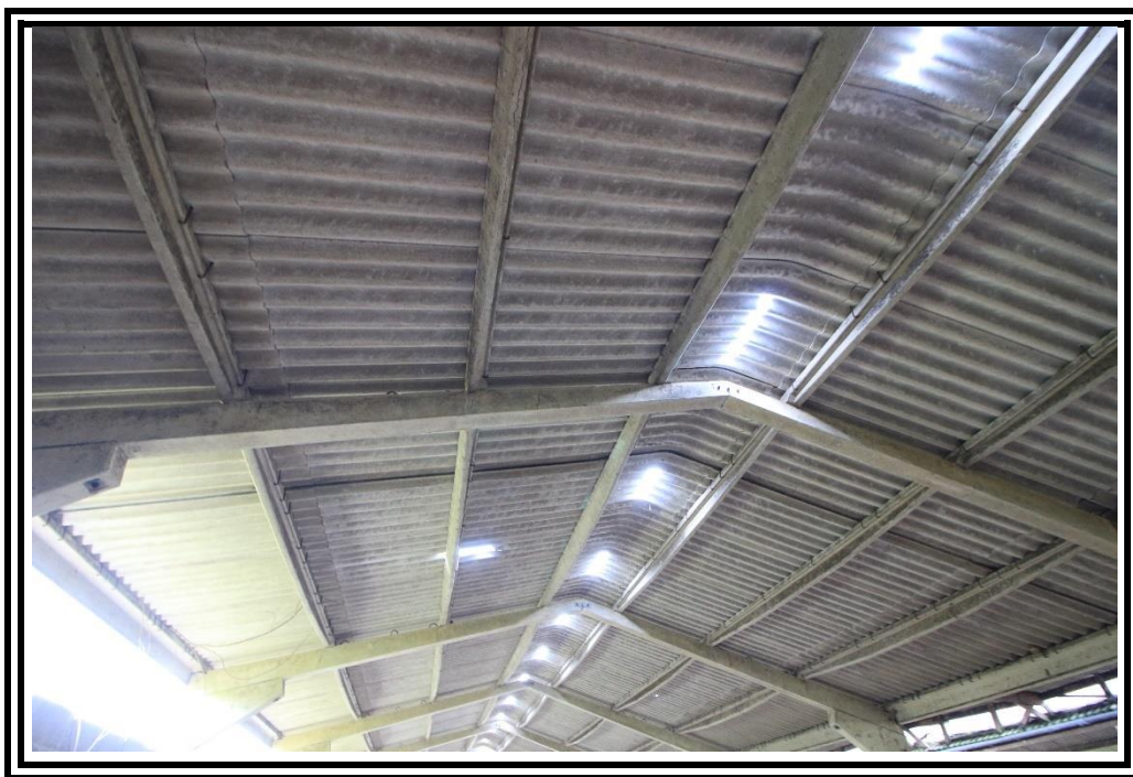
Photo 12: Building CD –internal view Part D
