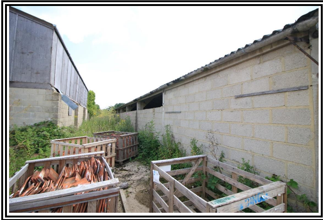
Photo 5: Building CD –Rear Elevation North Part C
