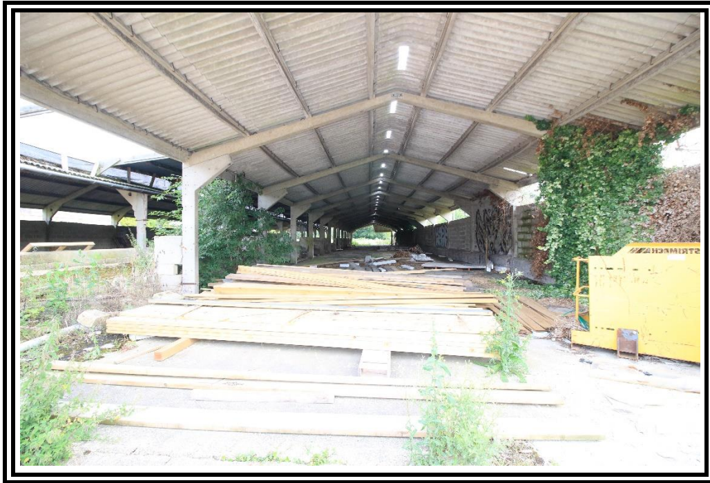
Photo 7: Building CD –internal view part D
