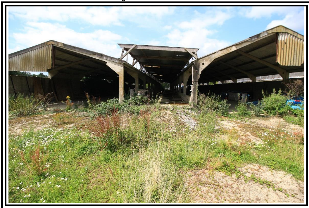
Photo 6: Building CD – Side Elevation East
