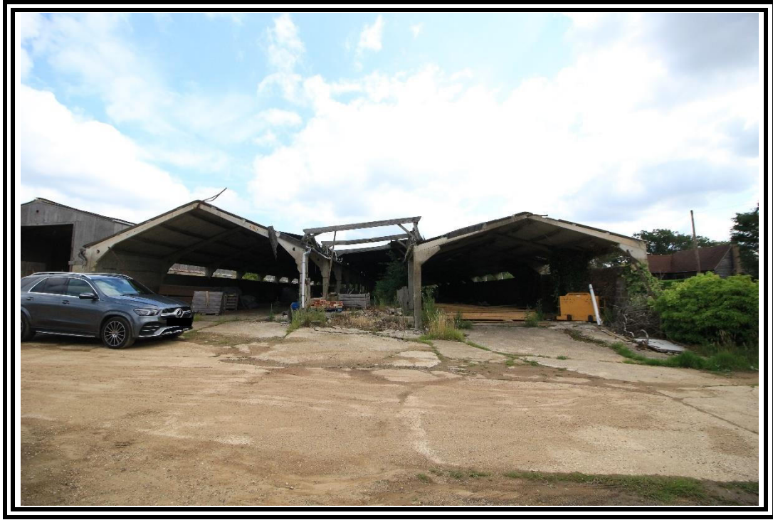
Photo 3: Building CD – Side Elevation West
