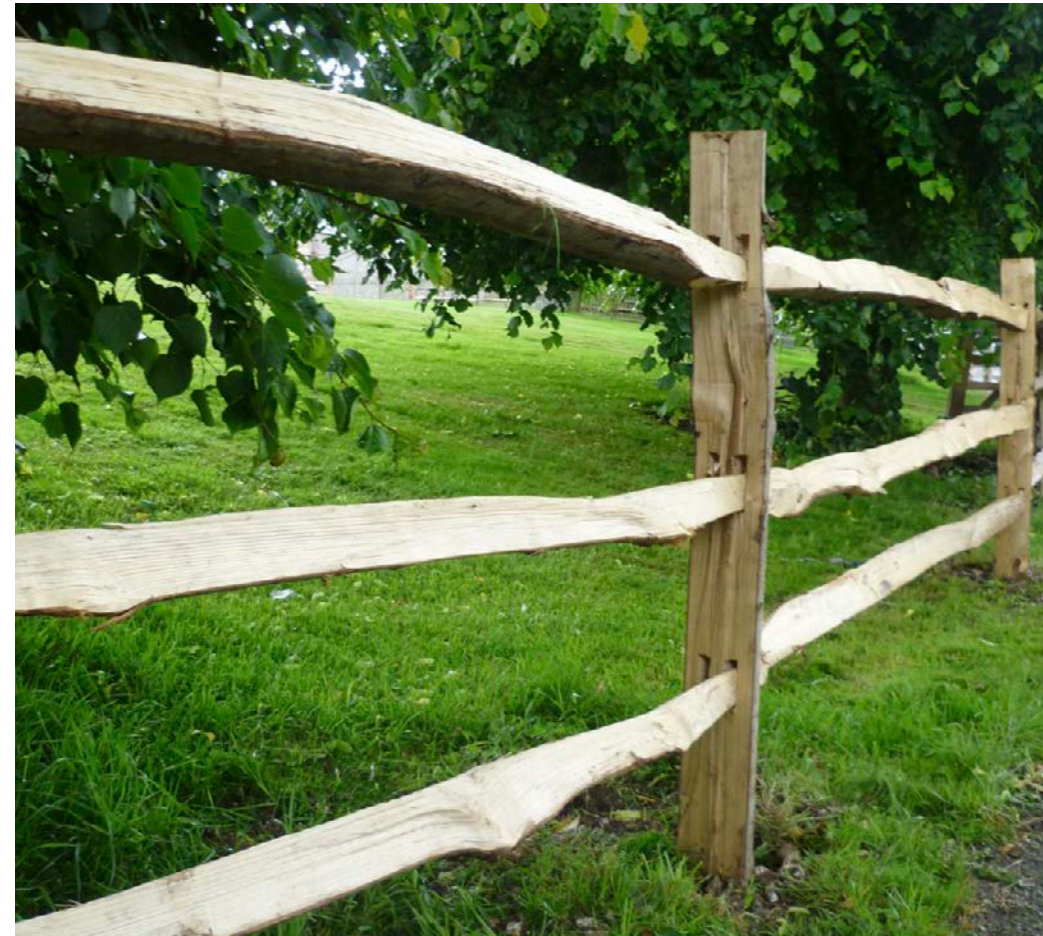
Cleft chestnut post and rail fencing
