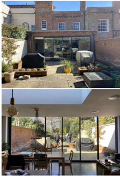
Figure 10 & 11 – Scarlett's Close Kitchen Extension External and Internal View
