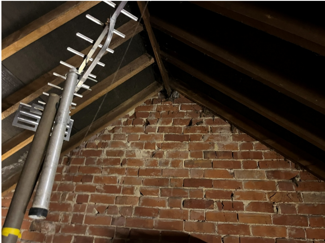
Figure 6. Loft looking west
