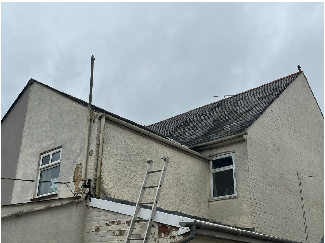
Figure 3. Southern and eastern elevations looking northwest
