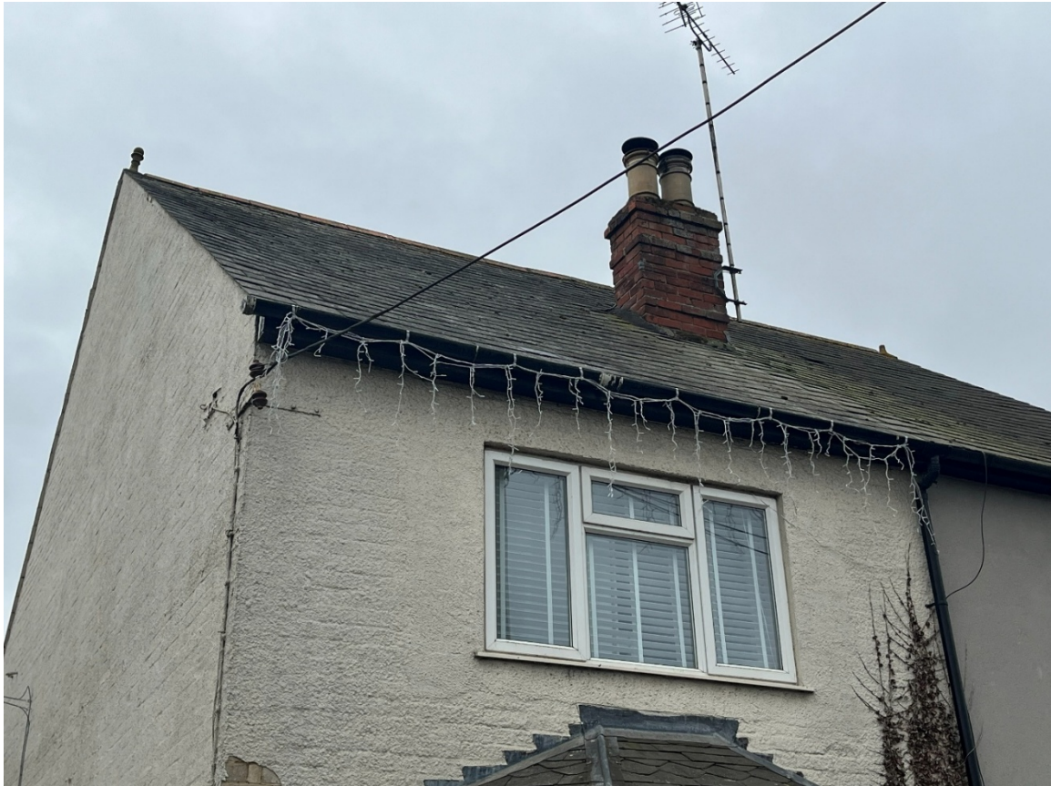
Figure 4. Northern and eastern elevations looking southwest
