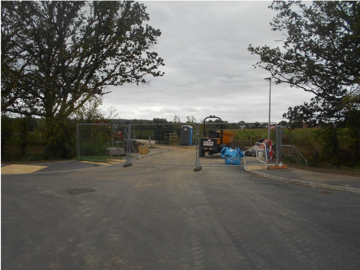
View looking south from the stub end of Shepherd Road on the existing development to the north of the audit site. This road will continue southward through the proposed new development, reaching Arborfield Road at the new access. The houses on Arborfield Road can just be made out in the distance
