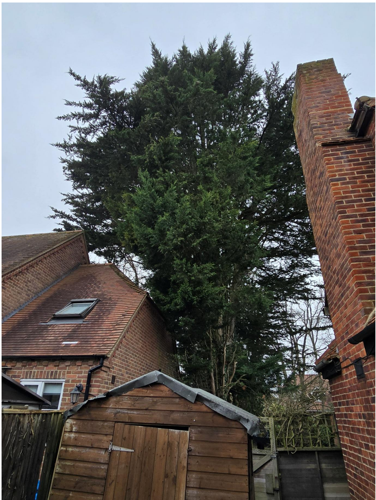
Photo 3) Branches close to neighbouring residential property.
