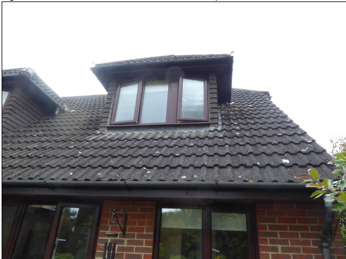
Figure 9. Dormer windows. 23b Pine Drive, Finchampstead, 02.07.24
