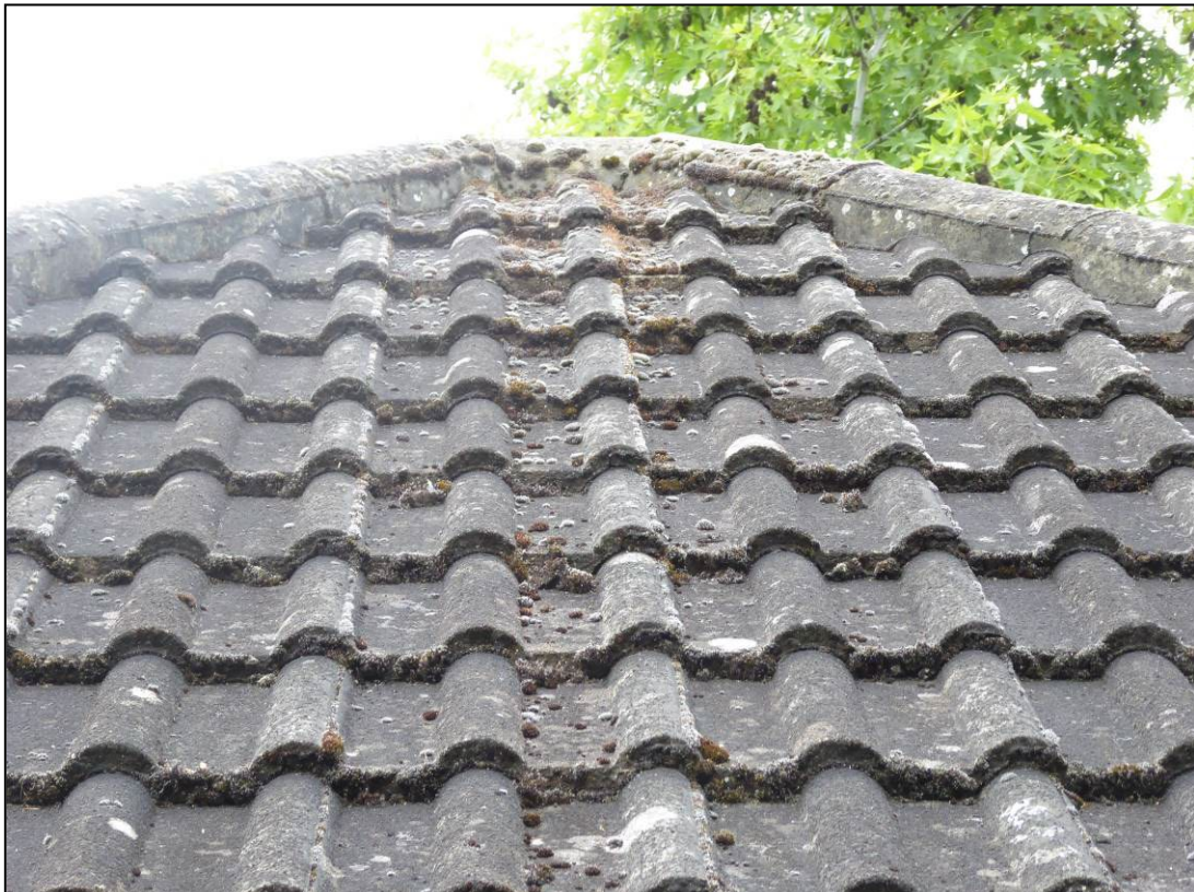
Figure 13. Roof tiles on detached garage. 23b Pine Drive, Finchampstead, 02.07.24
