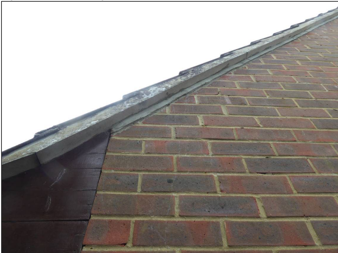
Figure 7. Example of verges. 23b Pine Drive, Finchampstead, 02.07.24
