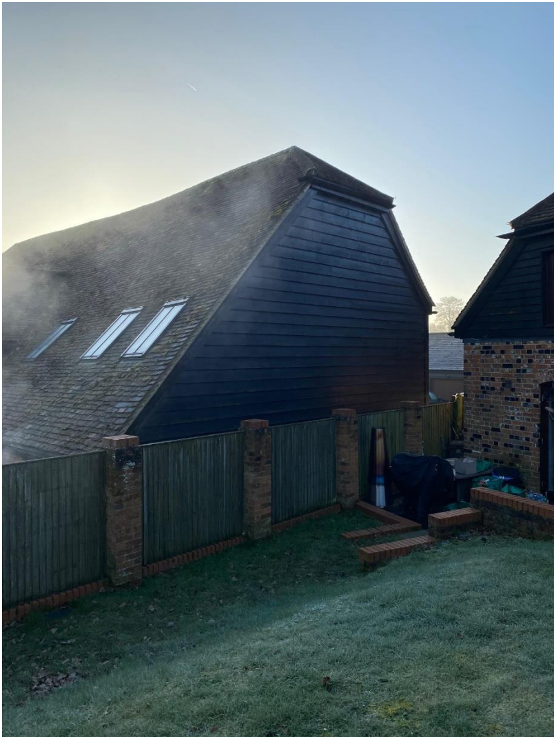
PIC 6. VIEW FROM GARDEN OF BARN 1
