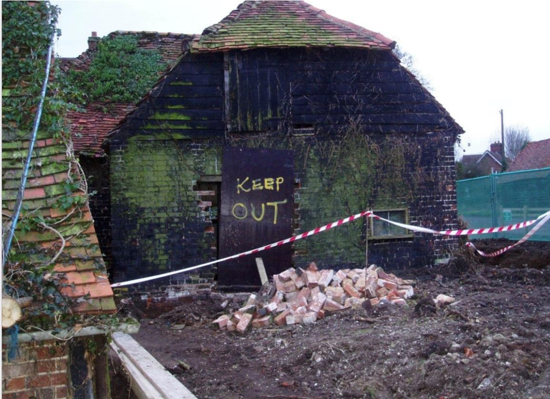
PIC 4. EXISTING BARN APPROX 2004. REAR ELEVATION
