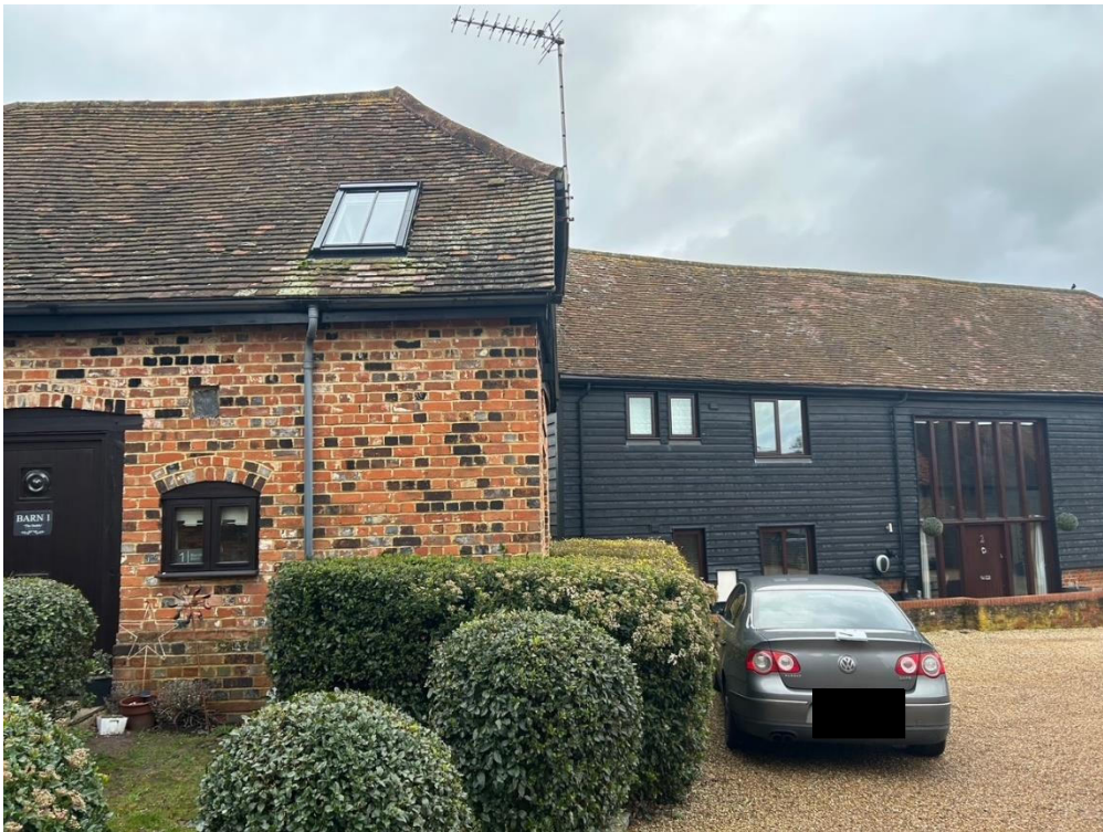
PIC 2. EXISTING FRONT ELEVATION SHOWING BARN 2
