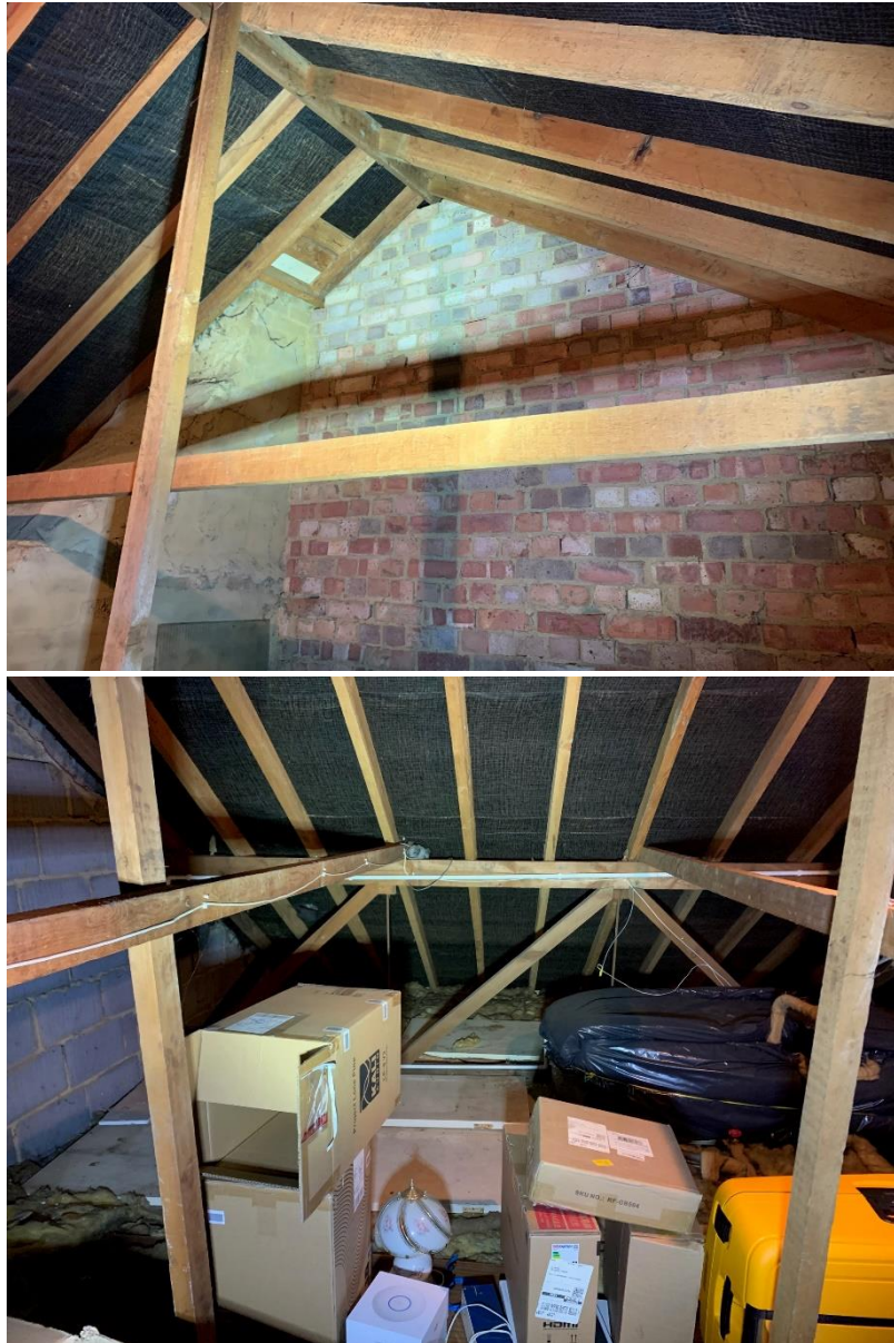
Plates 3-5 - Internal roof images
