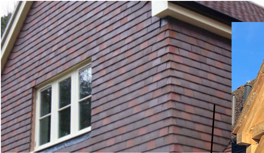
clay plain tile hanging Painted timber flush casement windows
