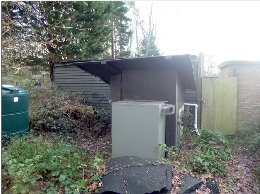
Photograph 3: Showing the rear of the buildings.
