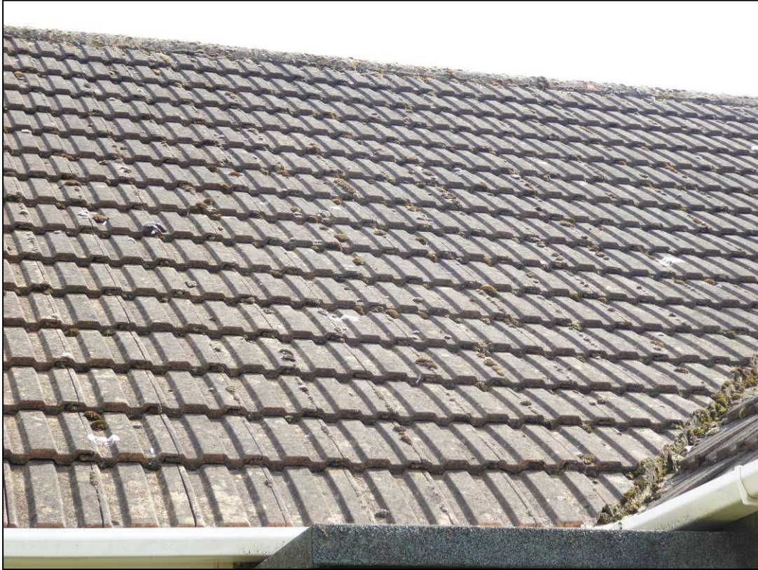
Figure 5. Tightly fitted roof tiles. 122 Victoria Road, Wargrave. 07.05.24
