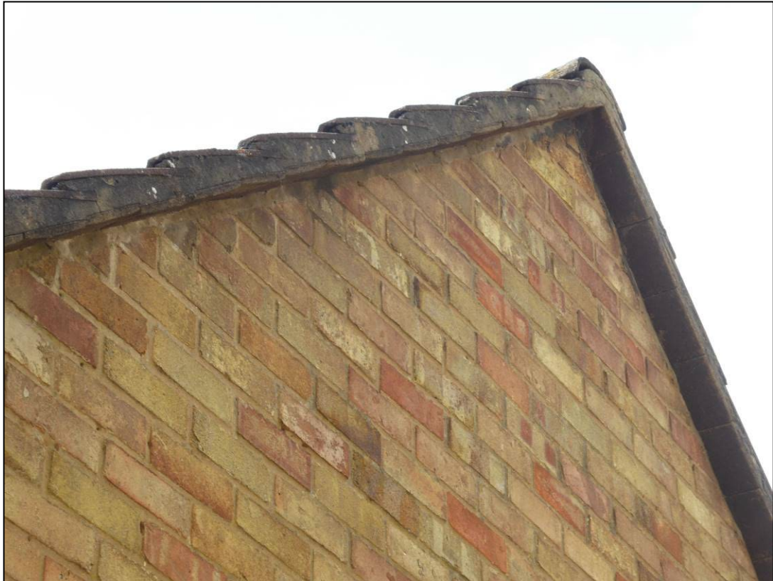
Figure 7. Example sealed verges. 122 Victoria Road, Wargrave. 07.05.24
