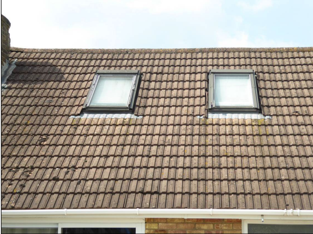
Figure 9. Tightly fitted lead flashing around Velux windows. 122 Victoria Road, Wargrave. 07.05.24
