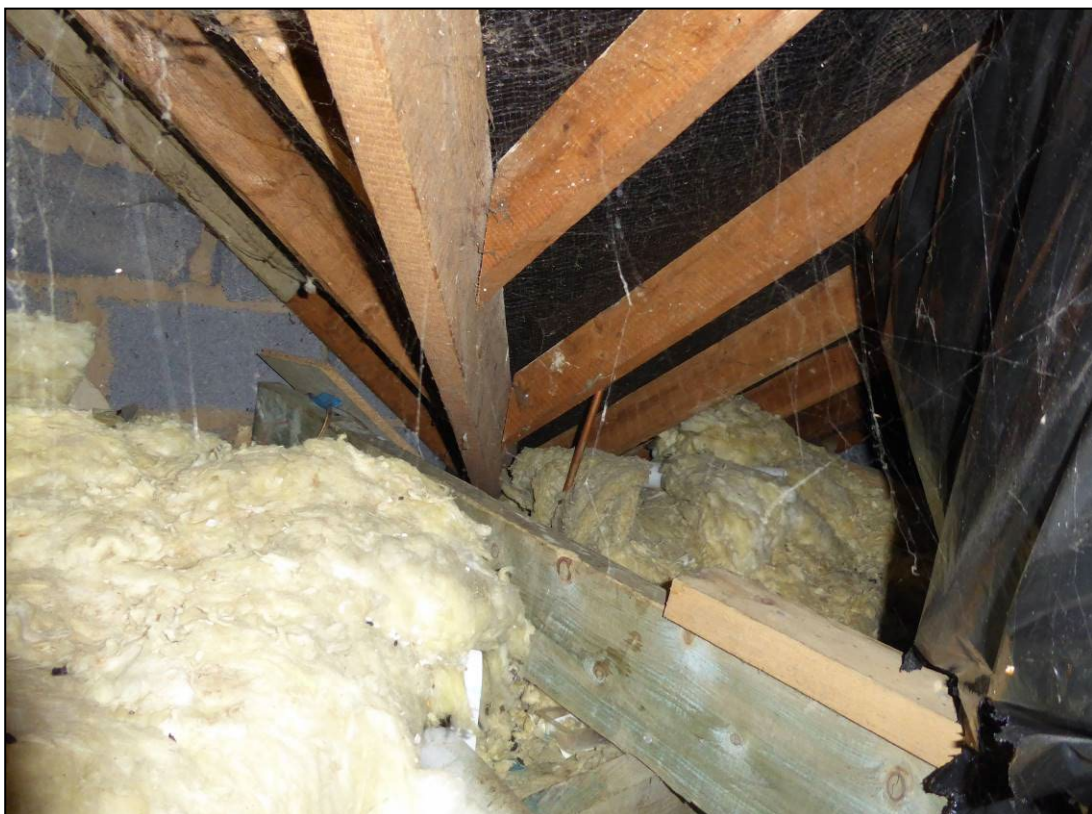
Figure 13. Example of under eaves storage cupboards. 122 Victoria Road, Wargrave. 07.05.24
