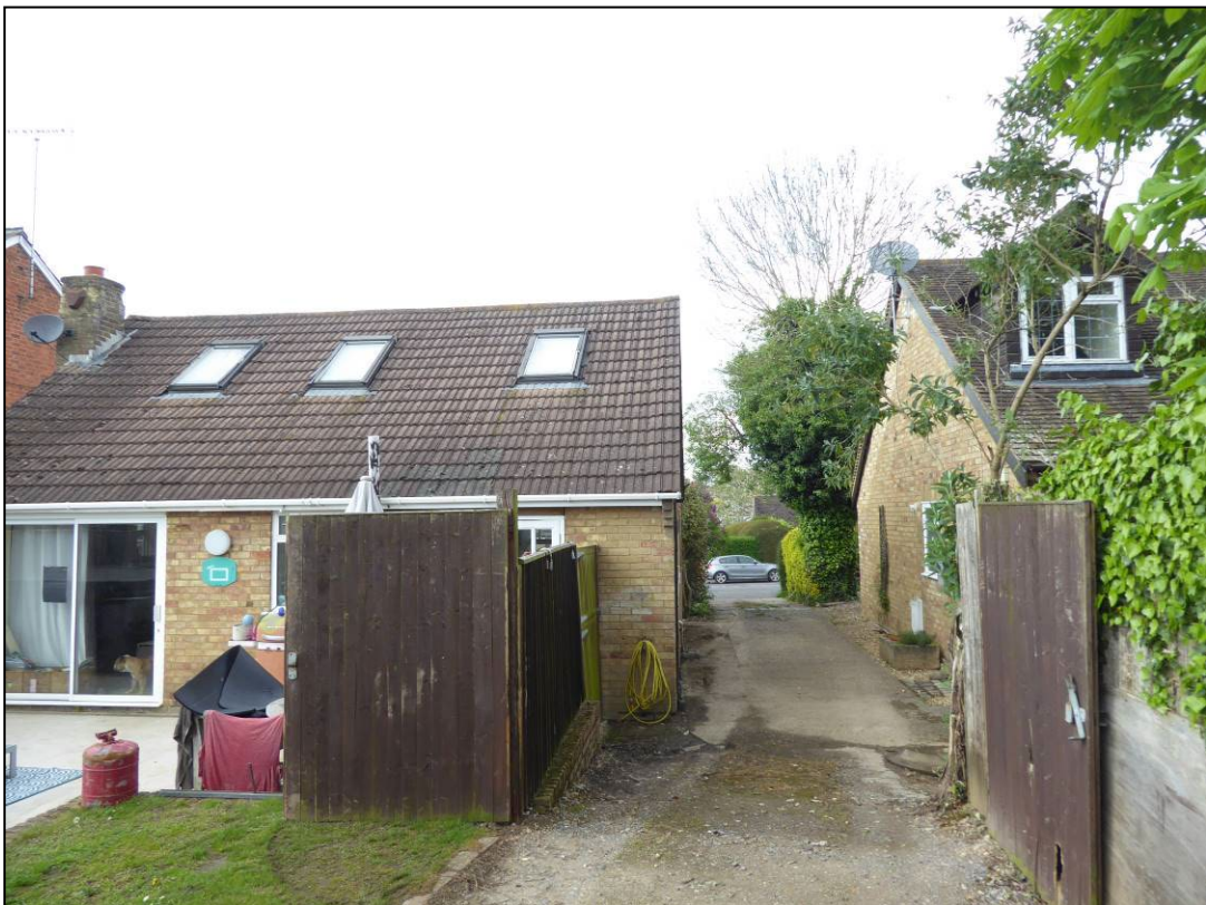
Figure 8. Velux windows. 122 Victoria Road, Wargrave. 07.05.24
