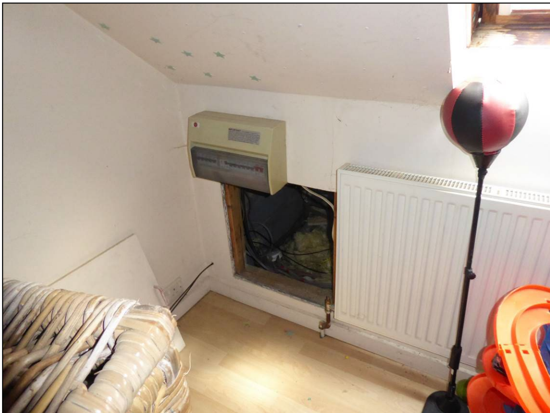
Figure 11. Example of hatch to eaves cupboard. 122 Victoria Road, Wargrave. 07.05.24
