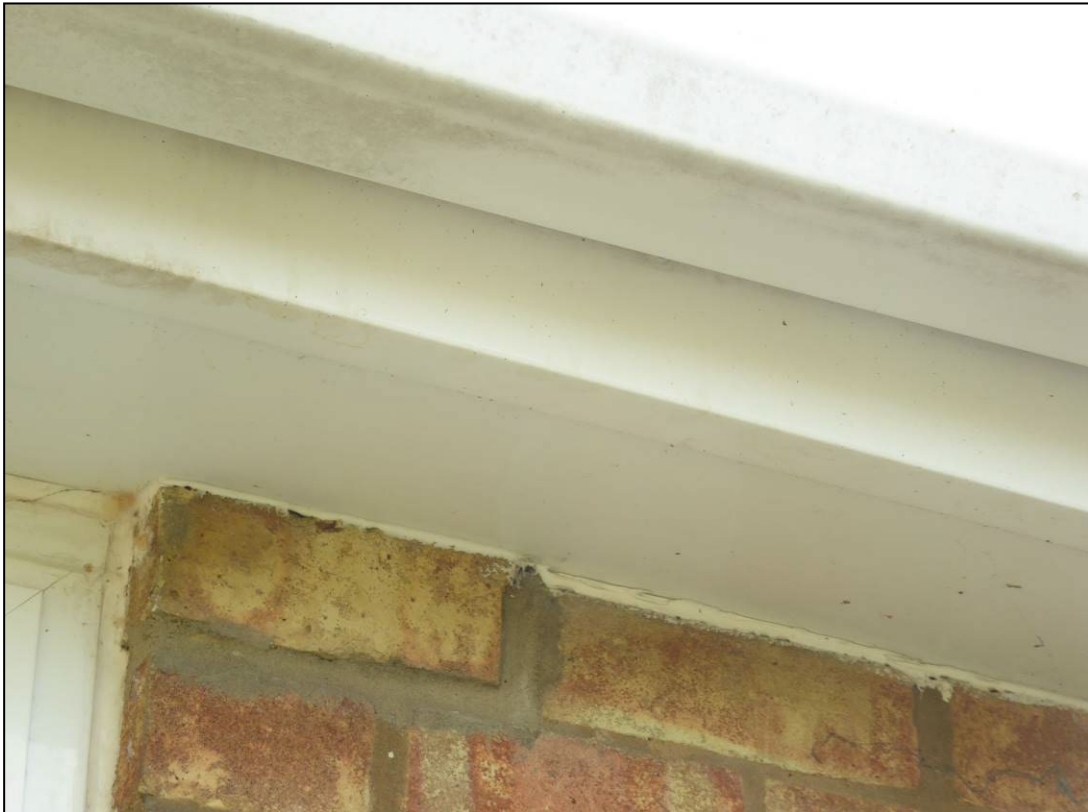
Figure 10. Soffits and fascia's. 122 Victoria Road, Wargrave. 07.05.24
