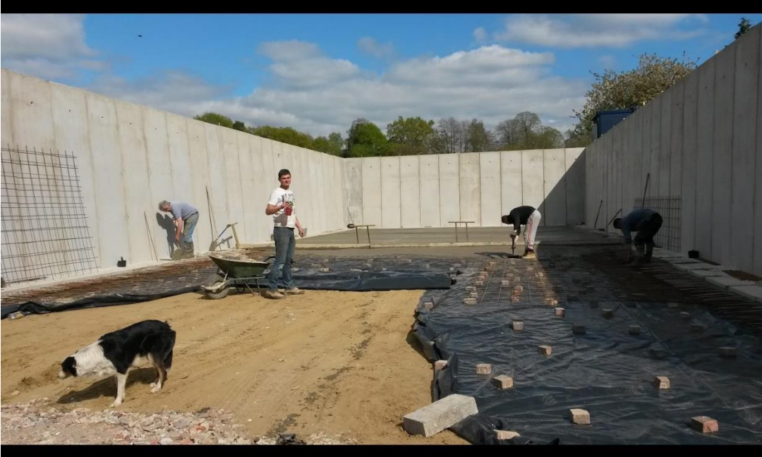
Photograph of Improvements to Silage Clamp (Previously Yard A) Dated 22 nd April 2015 and 9 th May 2015
