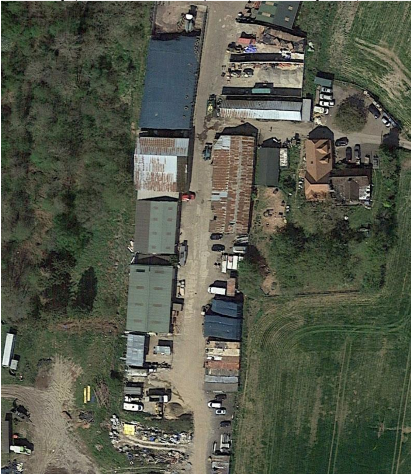
Aerial Photograph of Hill Farm dated 15 th April 2020 (Source – Google Earth)
