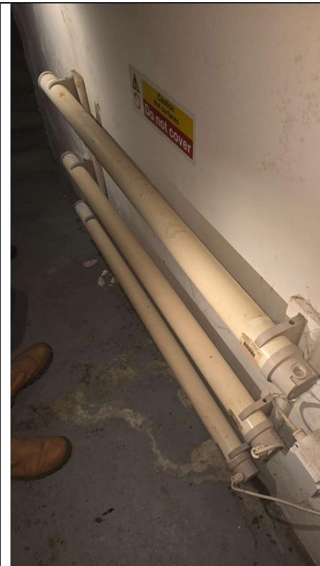
Fig 6 Existing heating pipework to be removed
