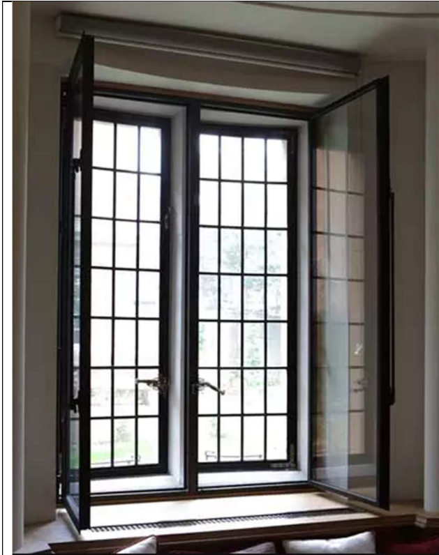
Fig 12 – Example of secondary glazing
