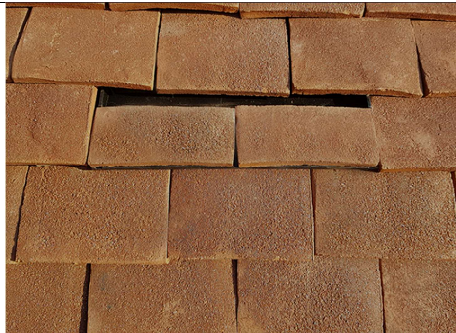
Fig 16 Example discrete tile vent by Klobber or Titan
