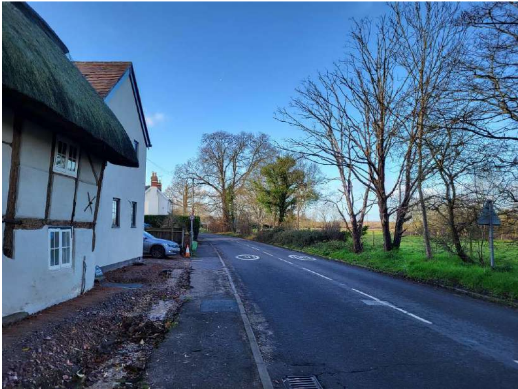
Plate 25: Parkers Cottage (December 2025, during works), with application site boundary to right
