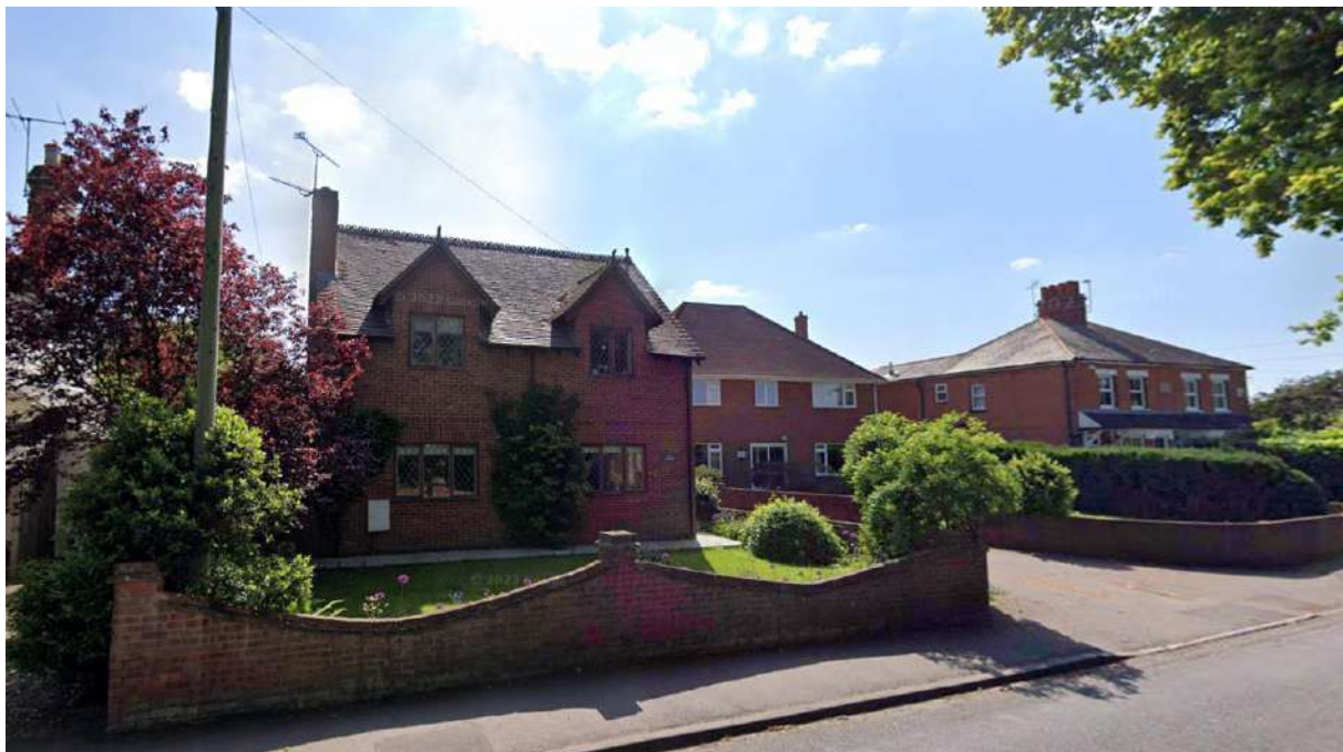
Plate 20: Late 20 th -century infill development to right (west) of Victoria House, with early 20 th -century Aylesford Villas to right beyond (Google, May 2023)
