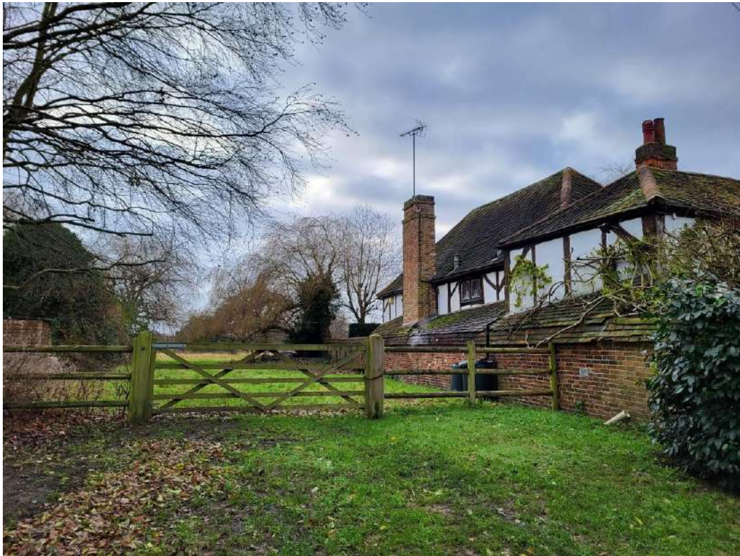
Plate 29: Extended side elevation of Elder Cottage, in context with adjoining historical field access
