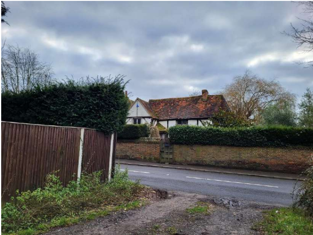
Plate 31: Elder Cottage as seen from the inset field gate to the application site
