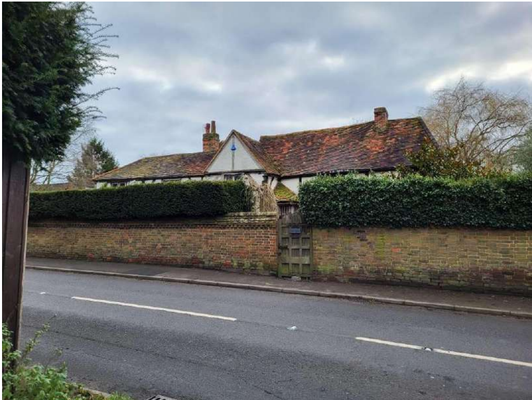
Plate 27: Elder Cottage as seen from Broadwater Lane in front of the field gate into the site
