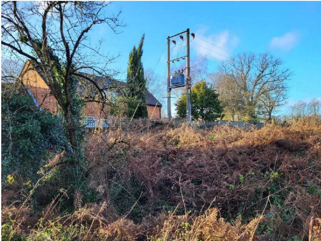
Plate 39: Looking across corner of site towards rear elevation of two-storey element of Long Barn
