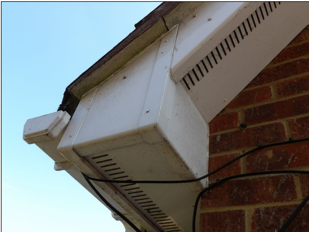
Figure 8. Example sealed soffits and fascias. 372 Barkham Road, Wokingham. 29.04.25
