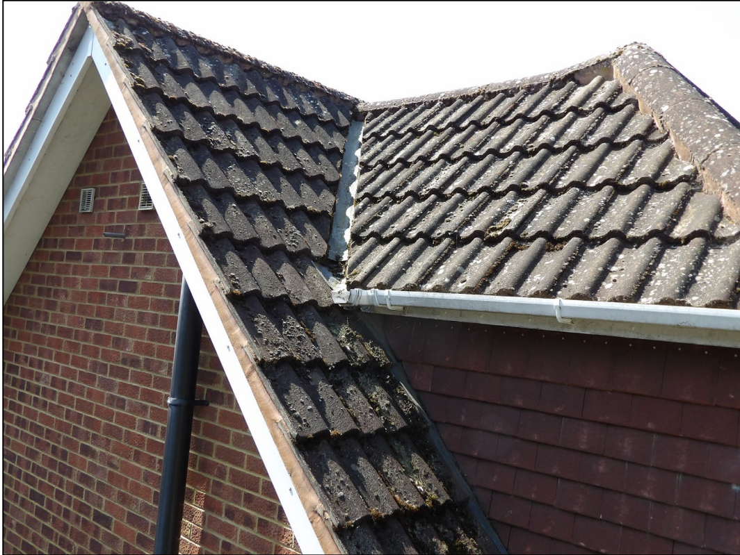
Figure 7. Example sealed verges. 372 Barkham Road, Wokingham. 29.04.25
