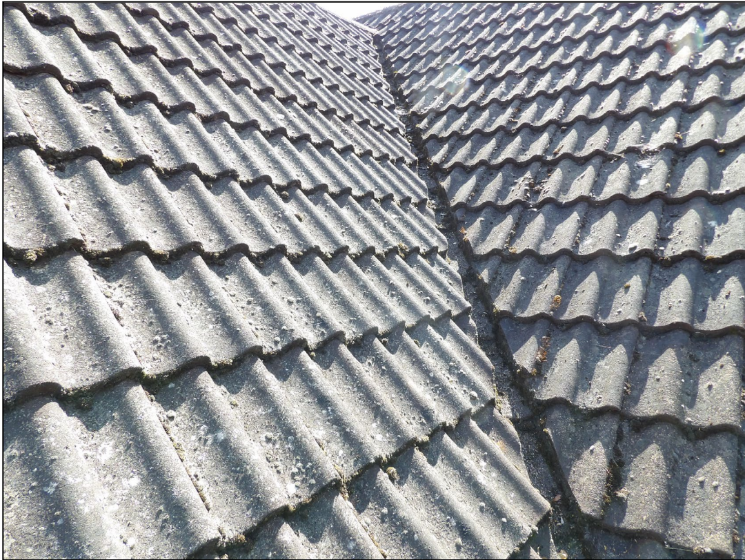
Figure 5. Example sealed roof tiles. 372 Barkham Road, Wokingham. 29.04.25
