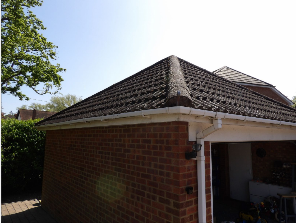
Figure 13. Well-sealed roof and hip tiles on garage. 372 Barkham Road, Wokingham. 29.04.25
