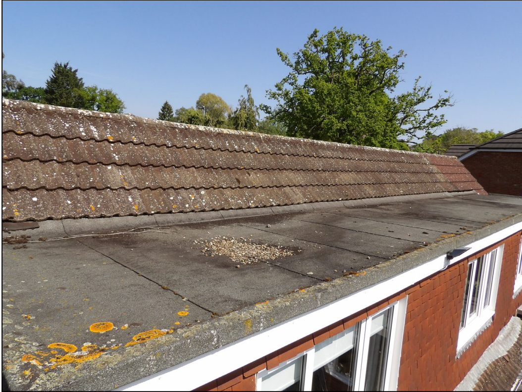
Figure 11. Bitumen roof of rear dormer. 372 Barkham Road, Wokingham. 29.04.25
