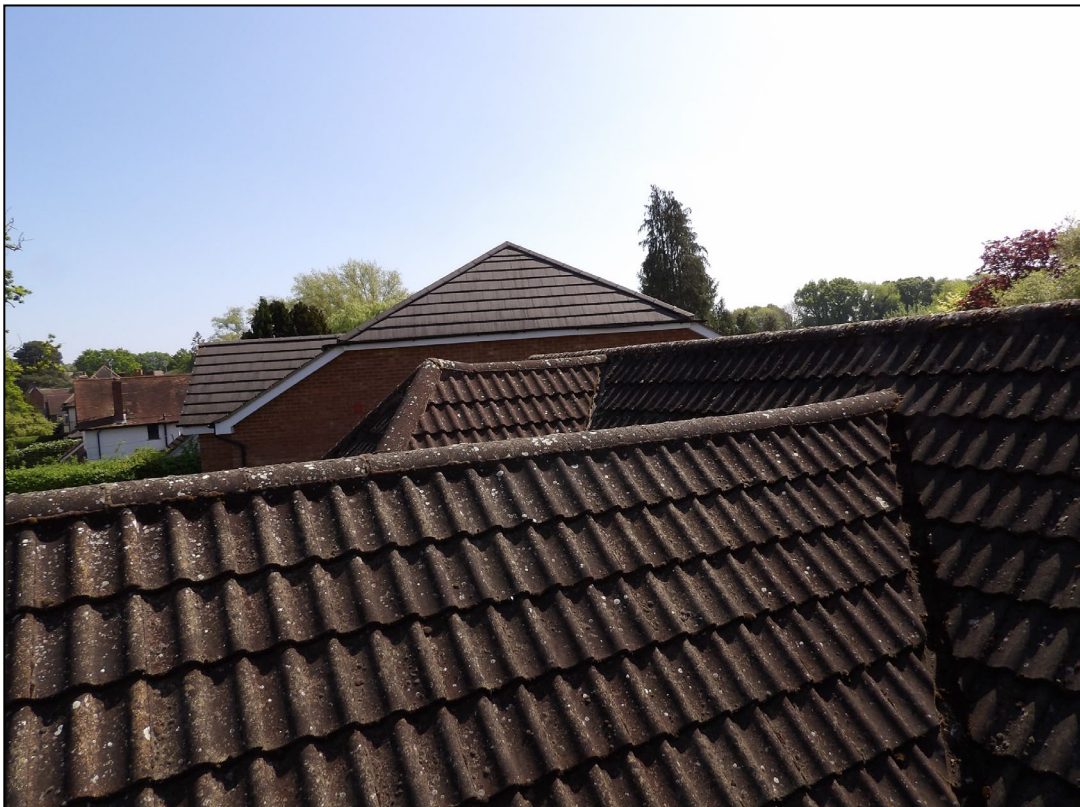
Figure 6. Example sealed ridge and hip tiles. 372 Barkham Road, Wokingham. 29.04.25
