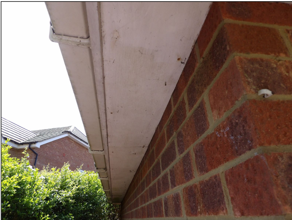
Figure 14. Example sealed soffits and fascias on garage. 372 Barkham Road, Wokingham. 29.04.25
