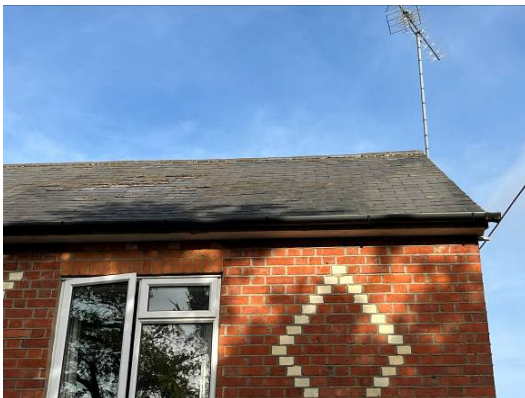
Photograph 3. Slate tiles sealed on roof and ridge (front elevation).
