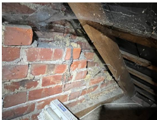
Photograph 15. Edges of the brickwork gables sealed by mortar (northeast eave space).
