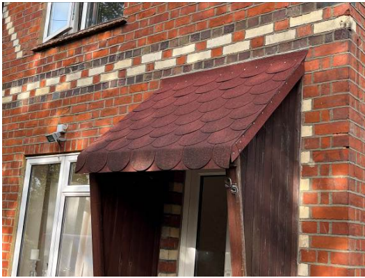
Photograph 5. Porch covered by a flat felt (front elevation).
