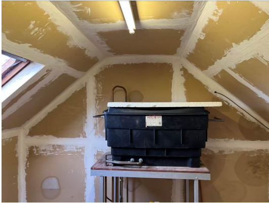
Photograph 11. Central roof void with plasterboard lining.
