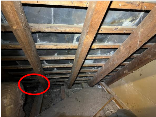
Photograph 13. Daylight within the eaves (southwest eaves space).
