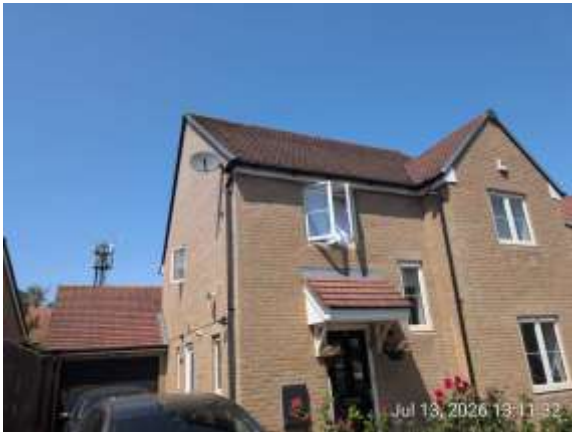
Building B1 southern elevation
