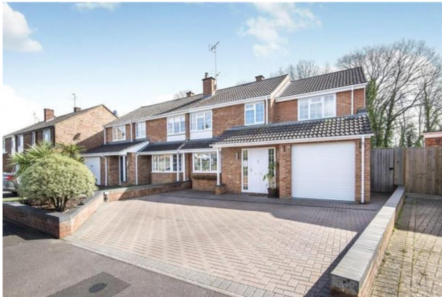
Before the Garage conversion – prior to November 2019 -
