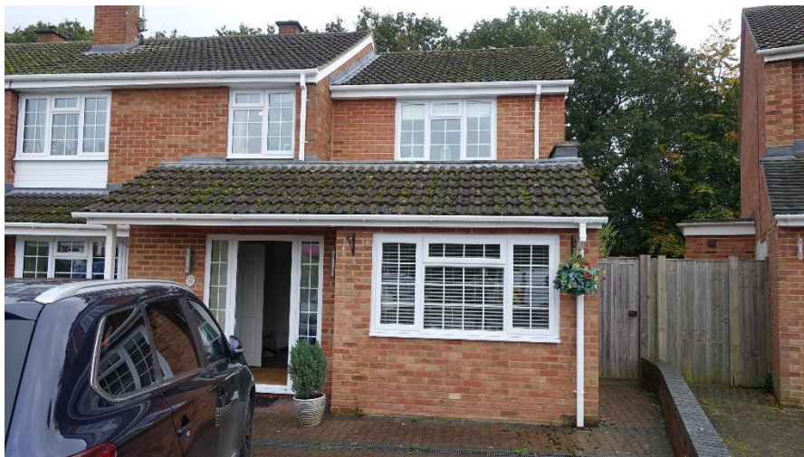
After Garage conversion – Following completion in February 2022
