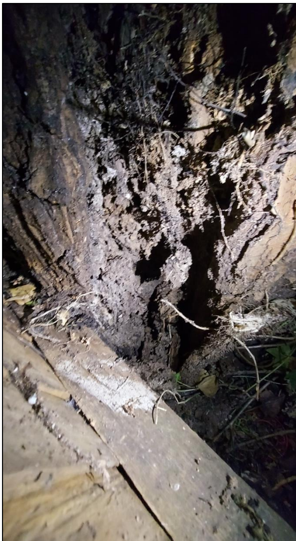
Photos 7 & 8: Decayed areas in lower trunk of T1.
