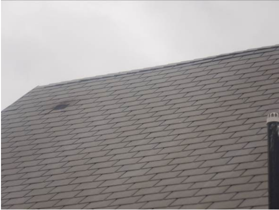
Photograph 3. Tightly fitted roof tiles (Rear elevation).
