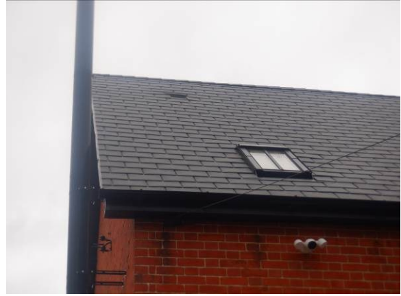
Photograph 4. Vents and skylights on the front roof elevation.
