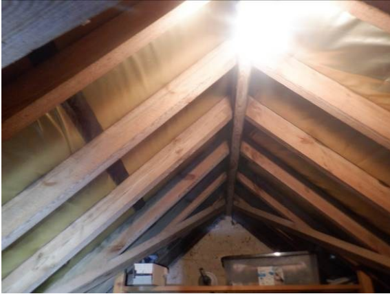
Photograph 8. Lined roof of cut and pitch construction with gold TLX BRM.
