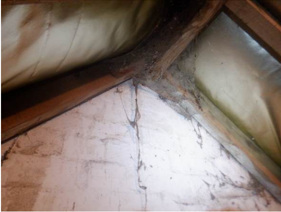
Photograph 12. Gable end of brickwork construction which was heavily cobwebbed.
