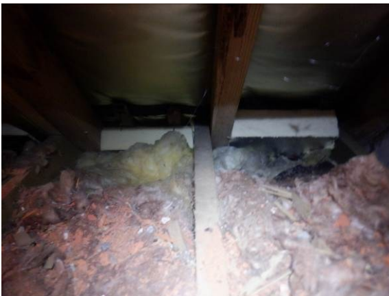
Photograph 11. Foiled covered insulation boards filling the eaves.
