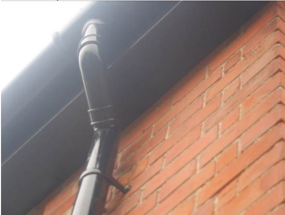
Photograph 5. Eaves tightly sealed with uPVC soffits.
