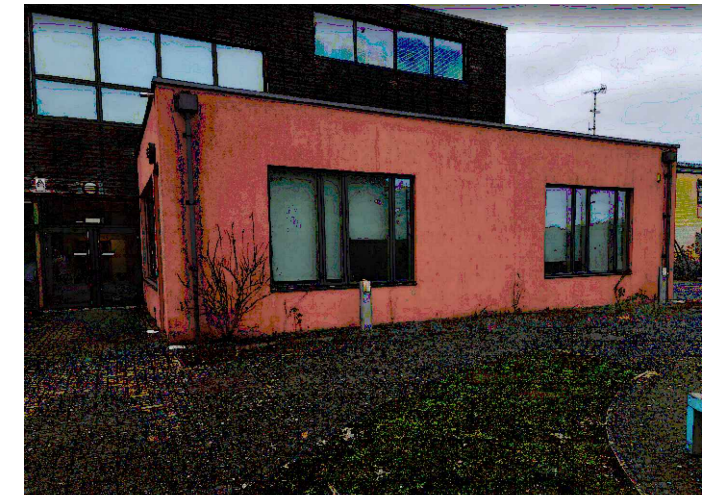
Image of Existing Building Opposite
