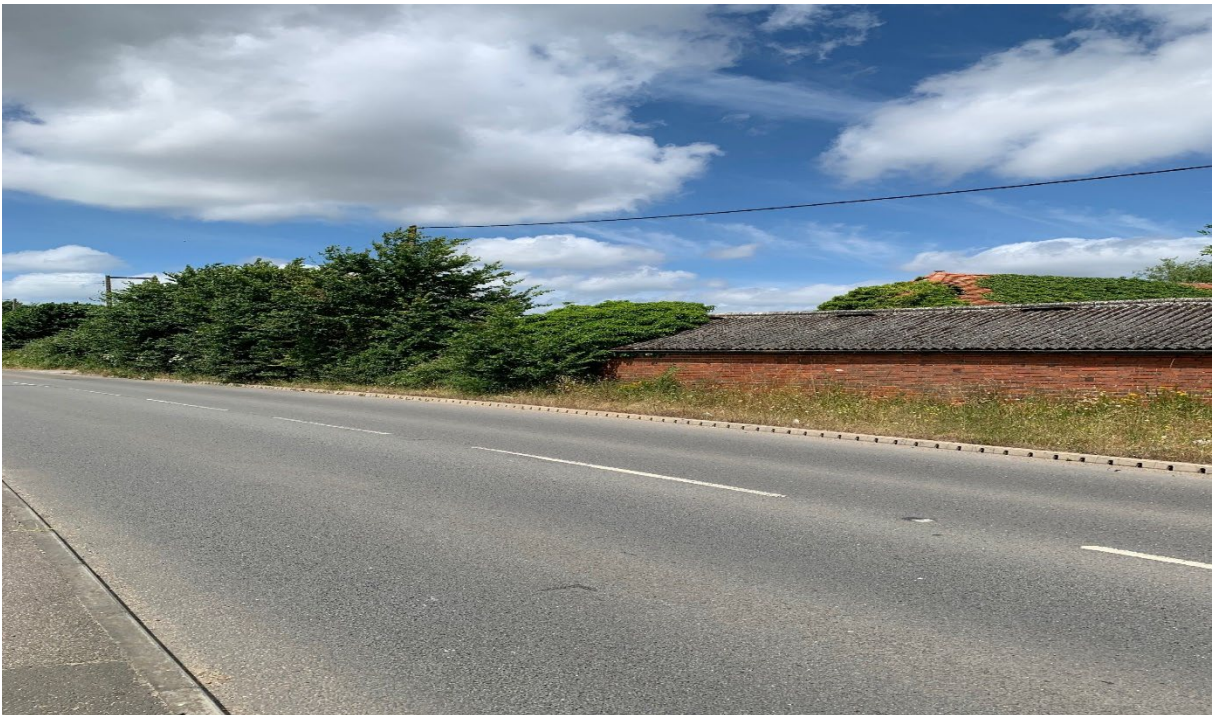
Image EDP A1.6: The barn within the south-eastern corner of the site, facing north-west viewed from the other side of the road.
