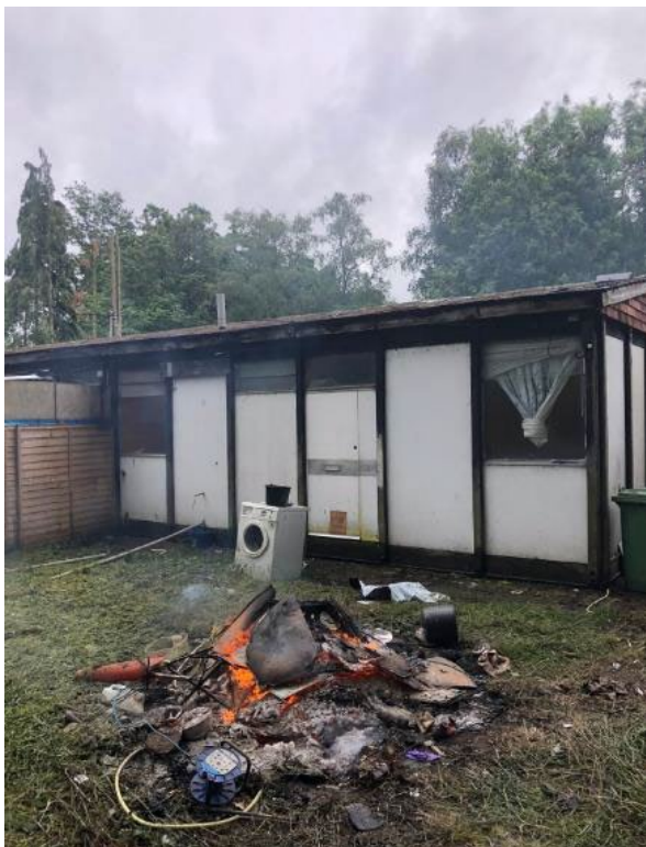
Photograph 11: rear garden of one of the dwellings, showing the burning of materials (including electricals)
