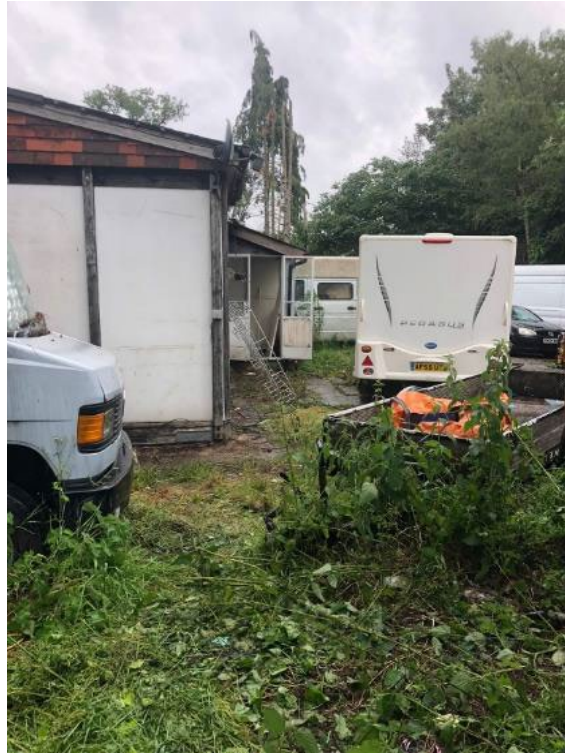
Photograph 6: south-western corner of the building (facing north-east)
