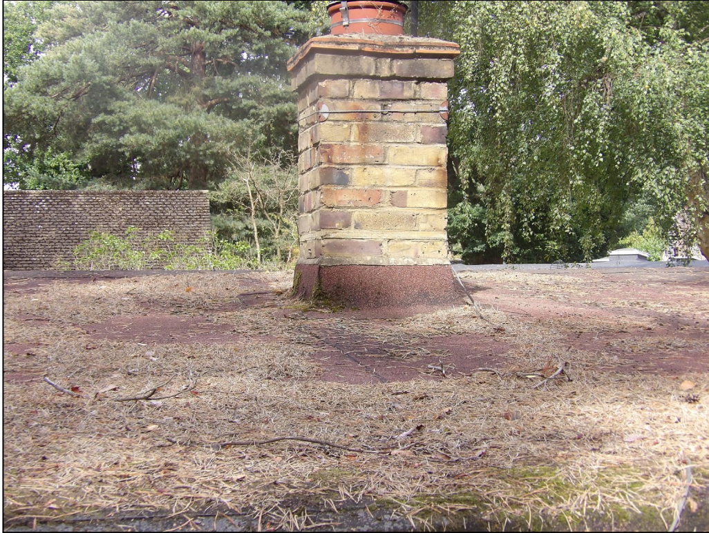
Figure 7. Example sealed bitumen felt around chimney stack. 4 Greenside, Crowthorne. 09.09.25
