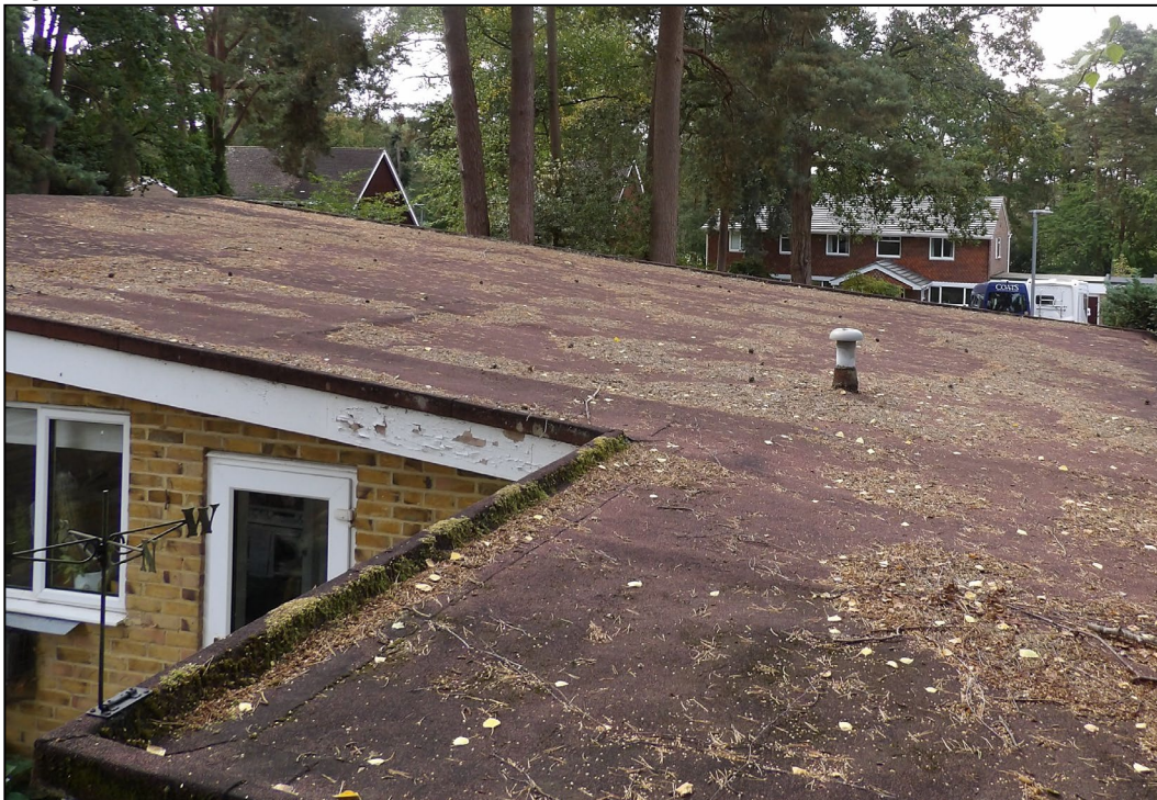
Figure 6. Example well fitted bitumen felt on roof. 4 Greenside, Crowthorne. 09.09.25
