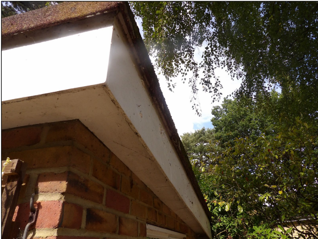
Figure 8. Example sealed soffits/fascias. 4 Greenside, Crowthorne. 09.09.25
