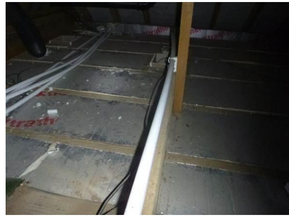
Photograph 21. Floor covered with foamboard insulation.
