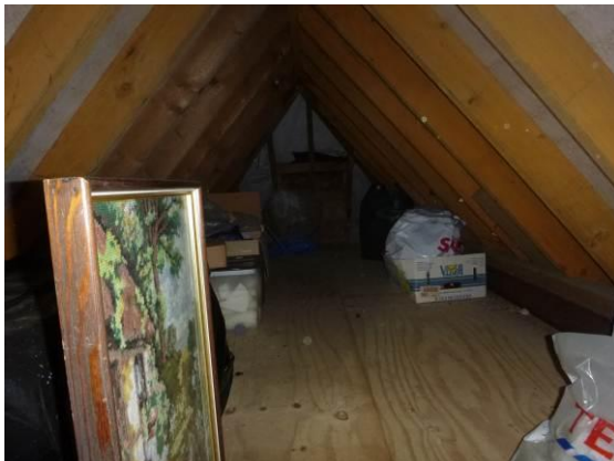
Photograph 12. Void 1 of cut and pitch construction approx. 1.75m in height.
