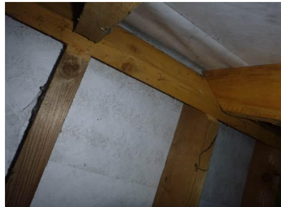
Photograph 13. Roof lined with intact breathable membrane, ridge beam lightly cobwebbed.
