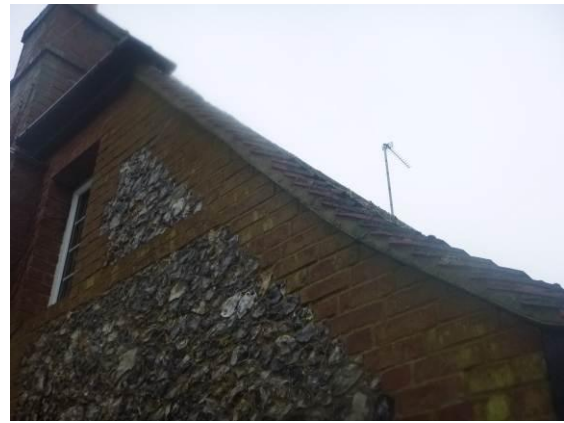
Photograph 6. Verge mortar intact.
