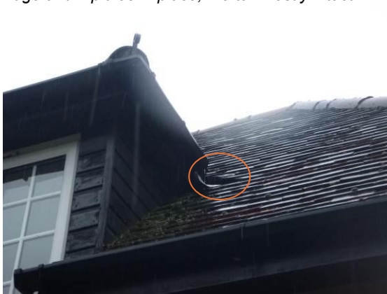
Photograph 7. Lifted tiles around dormers.
