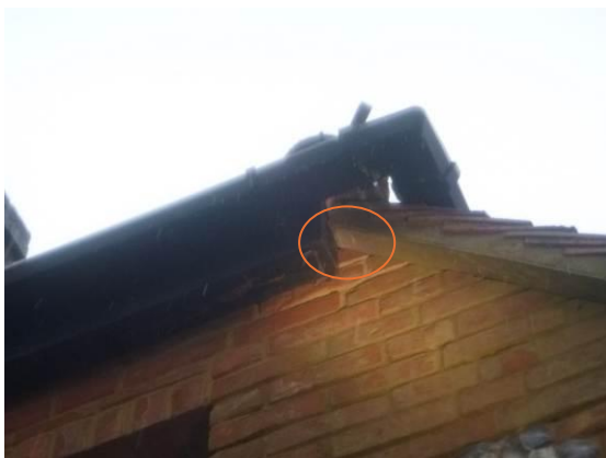
Photograph 9. Timber soffits with plastic mesh and occasional gaps.
