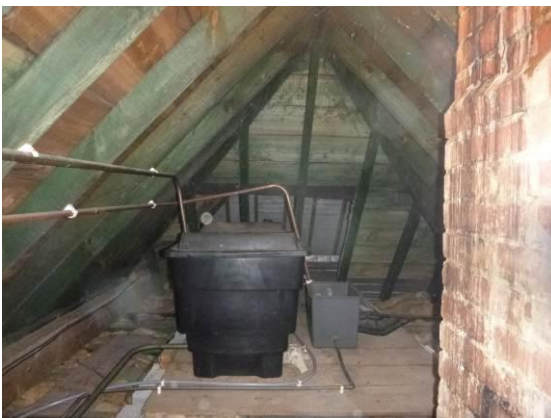
Photograph 18. Void 2 lined with sarking, fibreglass insulation on floor, boards in places.
