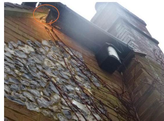
Photograph 10 Timber soffits with plastic mesh and occasional gaps.
