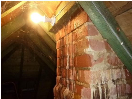
Photograph 22. Leaking southernmost chimney.
