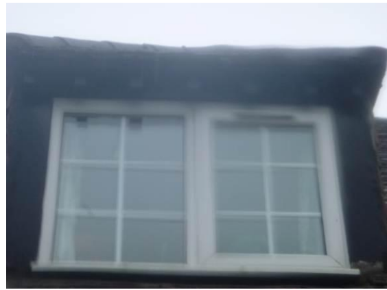
Photograph 11. Gaps behind hanging tiles on front gable end (front elevation); dropping stuck to glass although not visible in the photograph.
