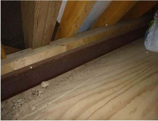
Photograph 14. Boarded floor with fibreglass roll and/or foamboard insulation underneath.
