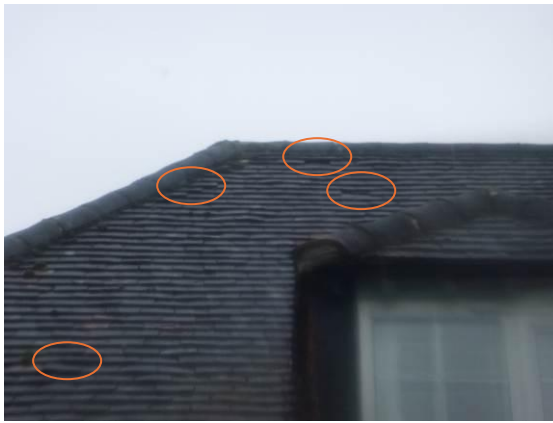
Photograph 5. Lifted and slipped tiles throughout, ridge and hip tiles in place, mortar mostly intact
