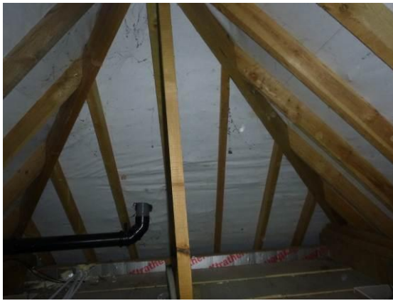
Photograph 20. Newer void area lined with breathable membrane with a small tear.
