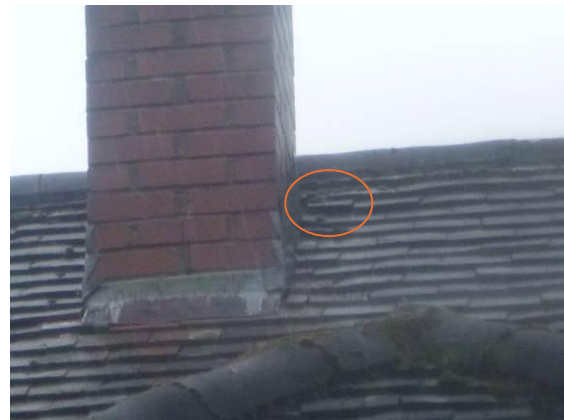
Photograph 8. Lifted tiles around southernmost chimney.
