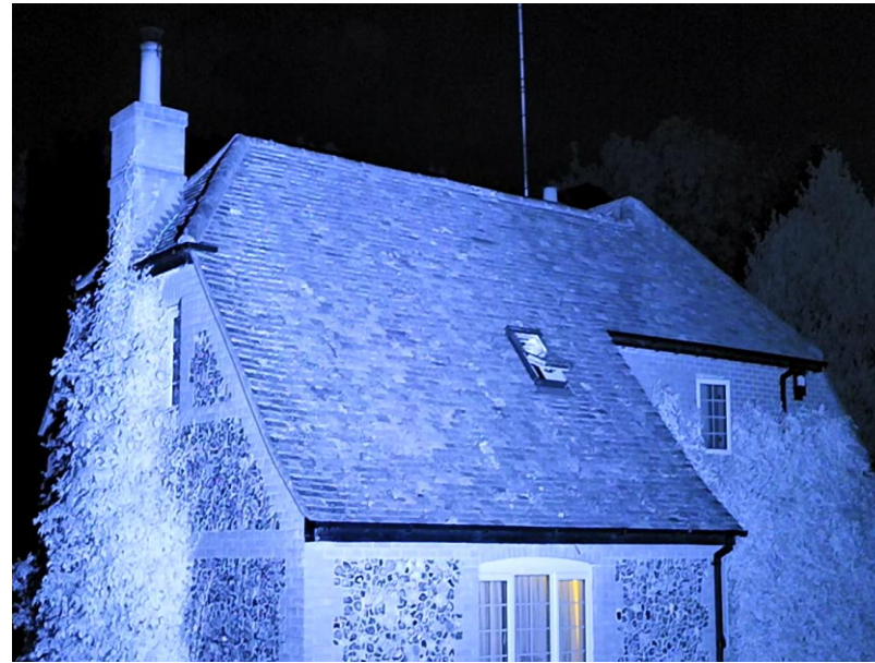
Sionyx Aurora Pro at Surveyor Location 2.
