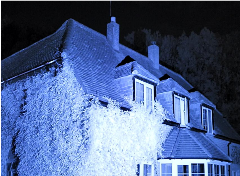
Sionyx Aurora Pro at Surveyor Location 3.
