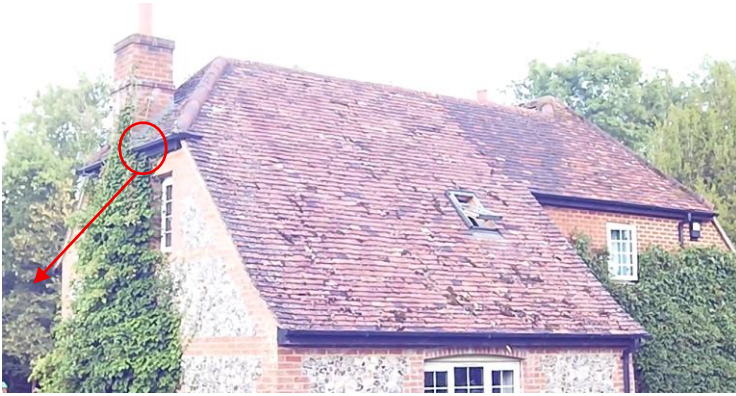
Photograph 5. Soprano pipistrelle emerging from eaves at 20:54 (Sionyx Pro surveyor at location 3)
