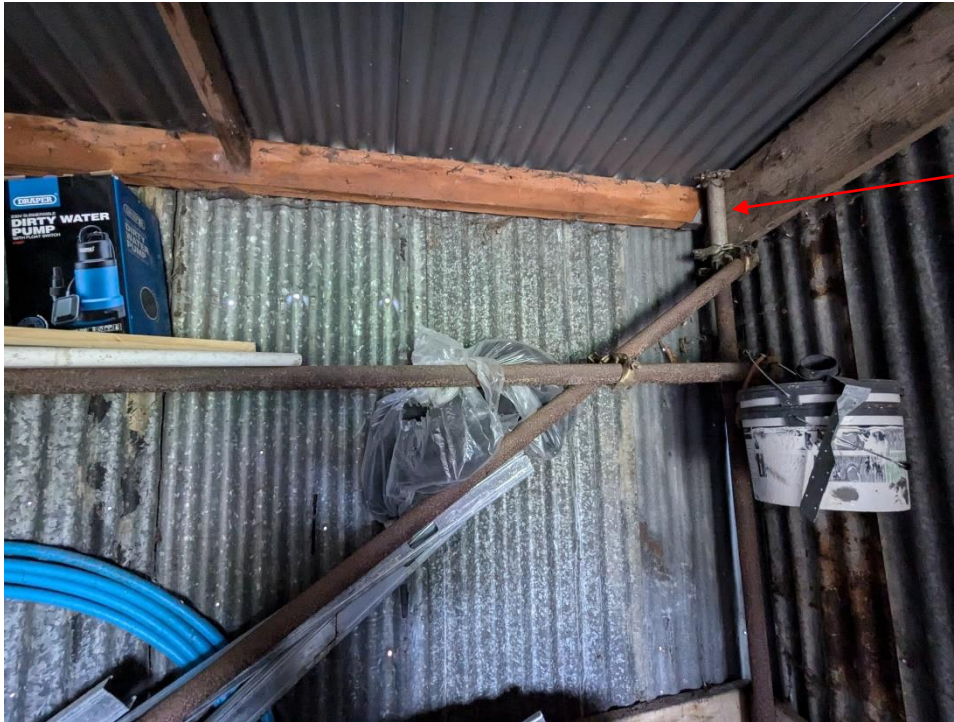
Photo 16 – Inclined scaffold brace at the rear of the structure.
