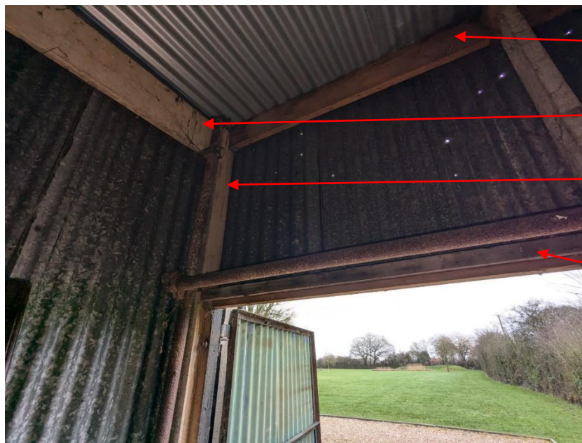
Photo 14 – Inside view showing the door structure and a vertical and horizontal scaffold prop.
