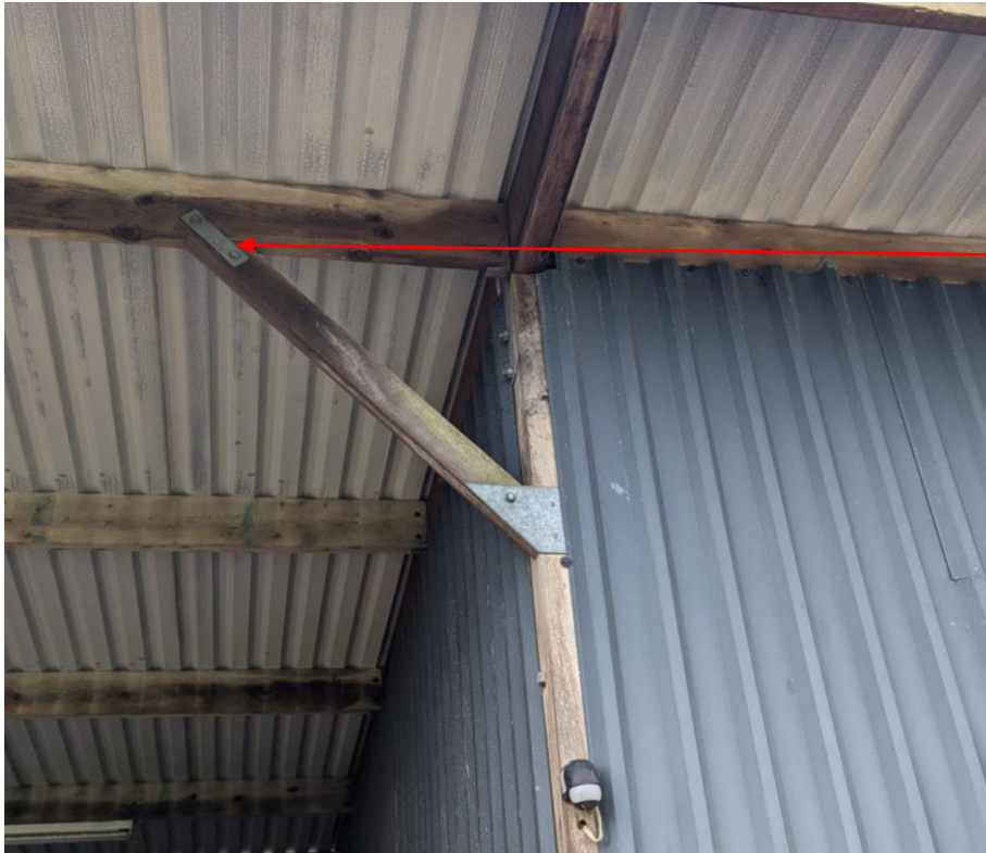
Photo 10 – Inclined strut to eaves beam
