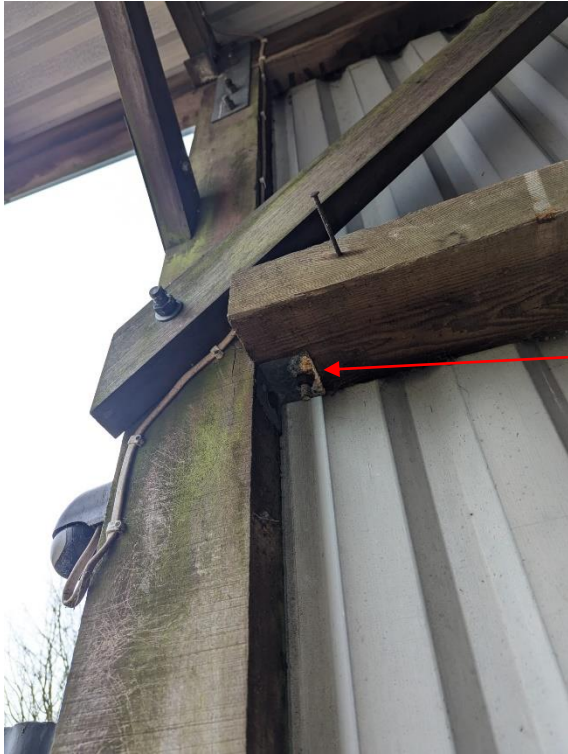
Photo 8 – Connection of the timber ring beam to post
