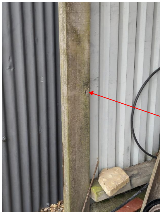
Photo 5 – Knotting of one of the timber posts
