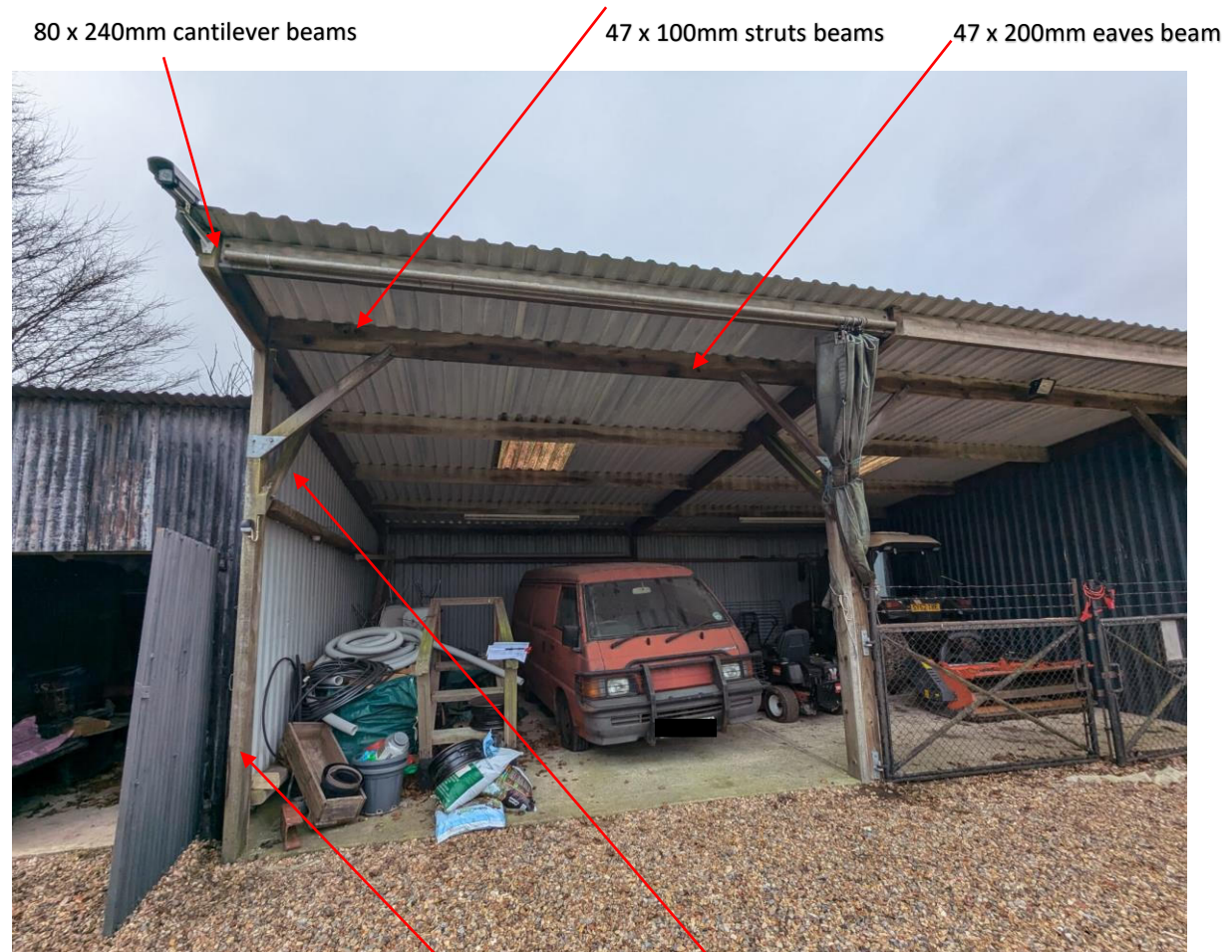
Photo 3 – Front elevation of the barn
