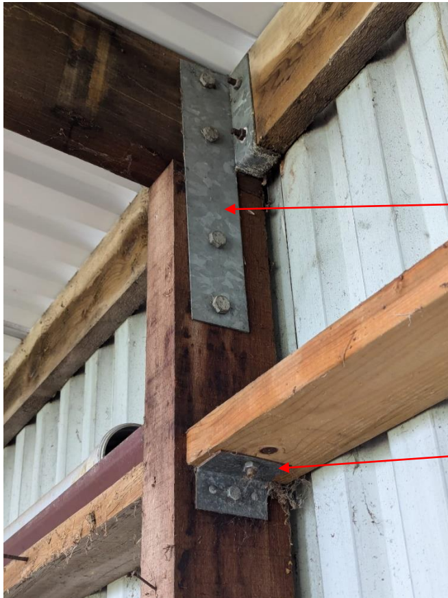
Photo 12 – Timber ring beam and cantilevered beam to rear timber post
