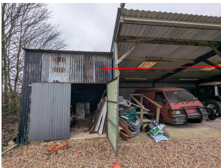
Photo 13 – Front elevation showing the storage structure constructed from timber and scaffolding
