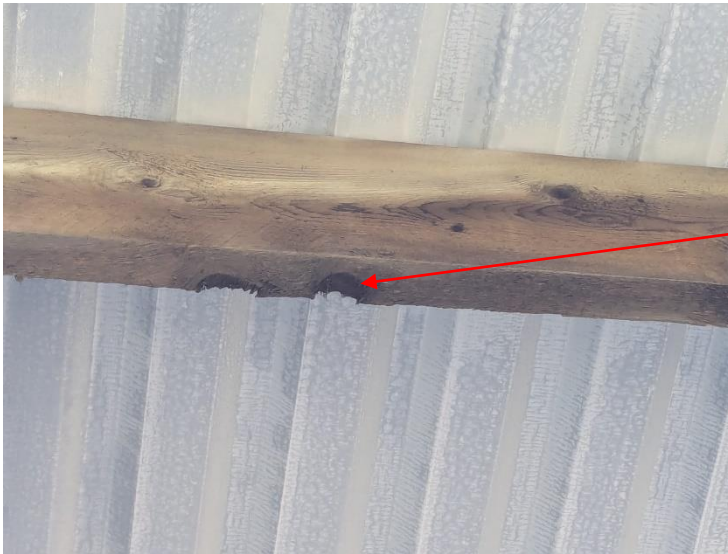
Photo 6 – Knotting/rotting of one of the timber edge beams
