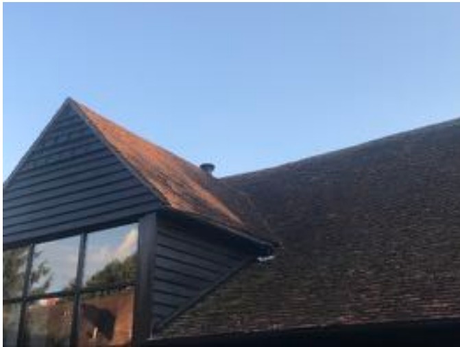
Image 1: Front of the roof being impacted (northeastern aspect)
