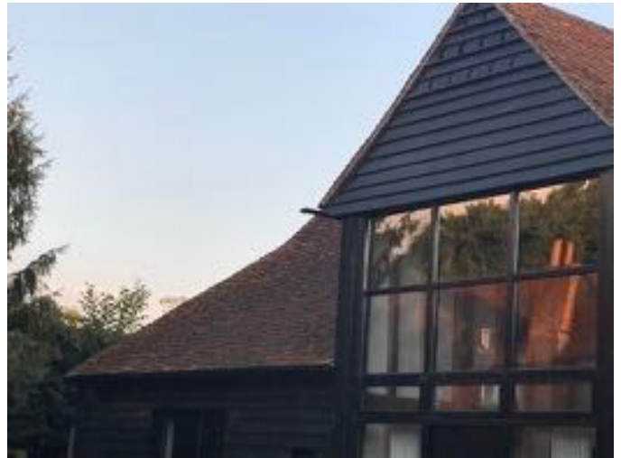
Image 2: Front of the roof being impacted (northwestern aspect)
