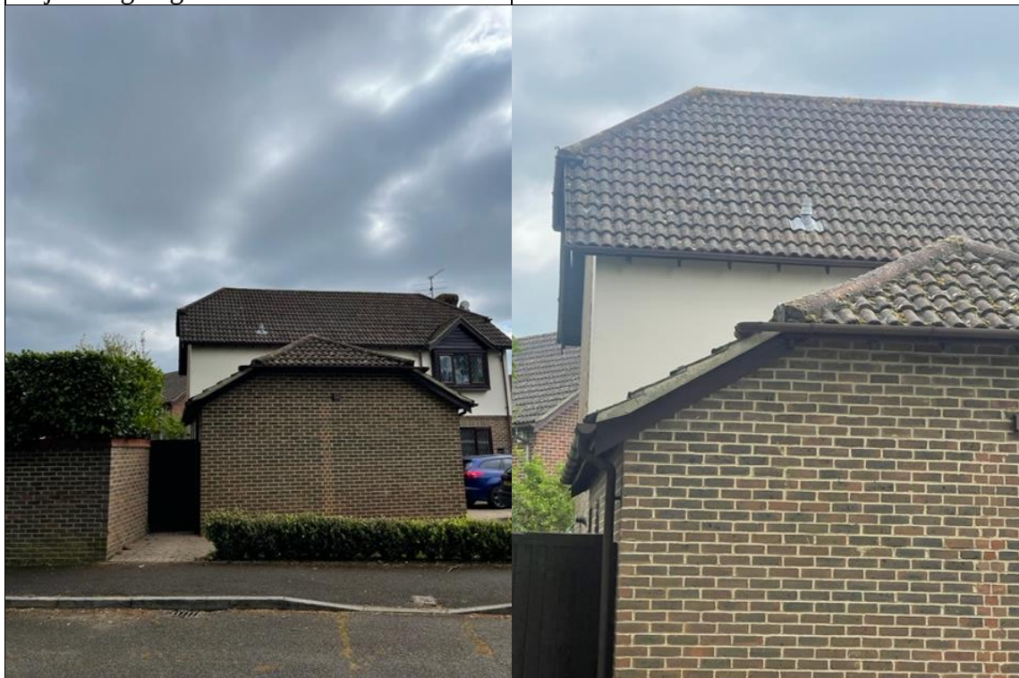
Photograph 3: Side of brick built garage.
