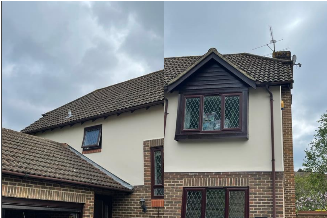
Photograph 1: Front elevation with adjacent garage
