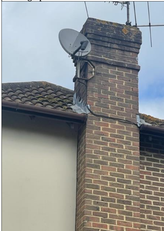
Photograph 7: Flashing around chimney.
