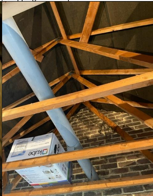
Photograph 20: Bitumen lined loft space.
