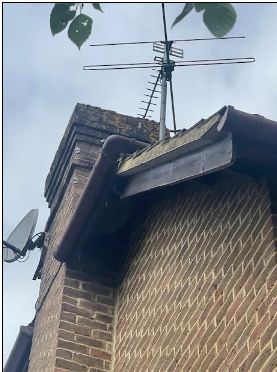
Photograph 9: Wooden barge board.
