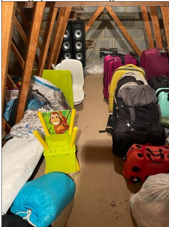
Photograph 11: Loft space used for storage.
