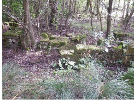
16. Remains of a brick wall within the woodland (TN4).
