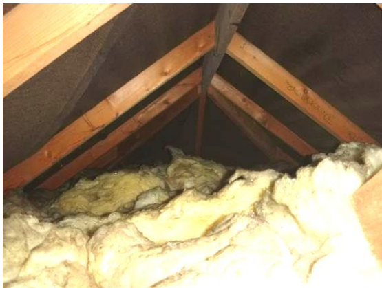
Photograph 22. Dormer void with intact bitumen felt and fibreglass insulation.
