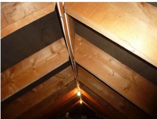
Photograph 20. Small roof void with intact liner and cobweb free ridge beam.
