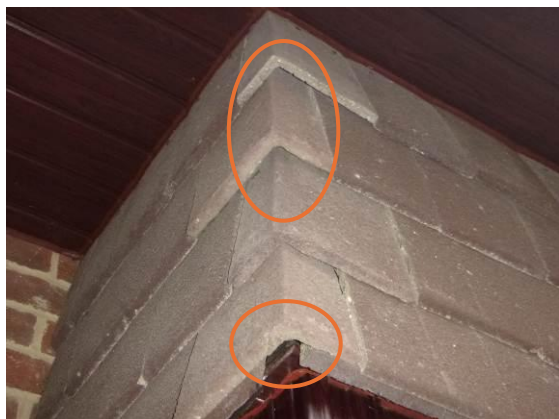
Photograph 14. Gaps behind hanging tiles above bay window ( TN6 ).
