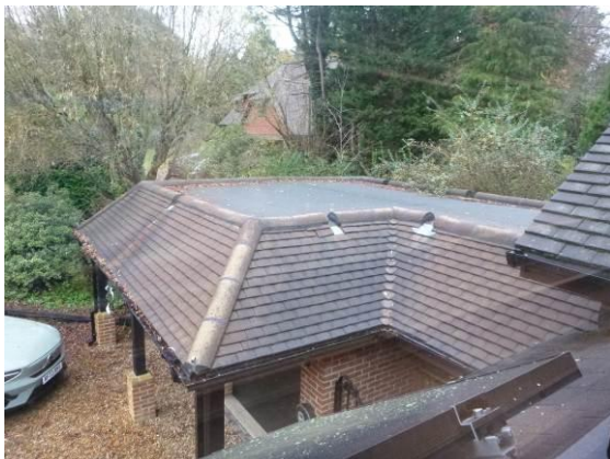
Photograph 7. Flat tiles on mansard roof of linked garage.
