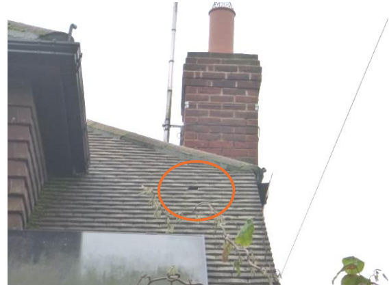
Photograph 4. Missing/broken roof tile (front elevation; TN1 ).
