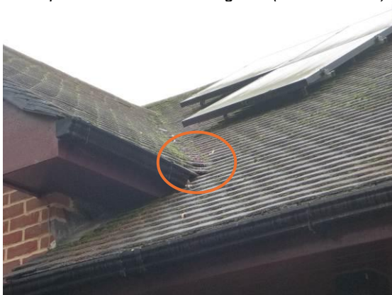
Photograph 5. Small gaps under lower valley tiles (front elevation; TN2 ).
