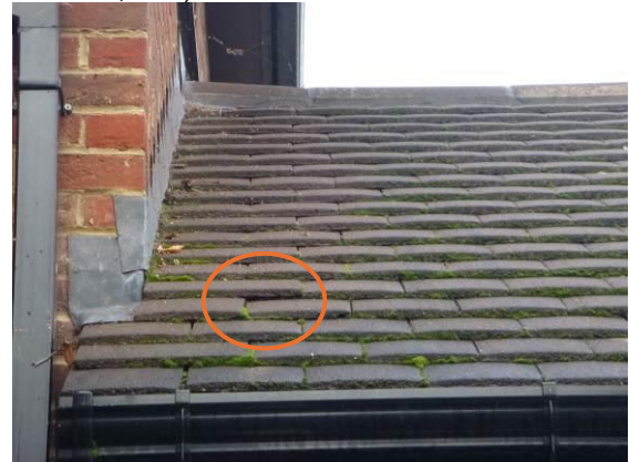
Photograph 6. Slight gap under lifted roof tile (rear elevation).
