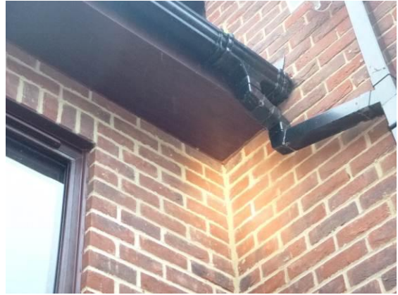
Photograph 19. Soffits tight to brickwork (rear elevation).
