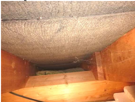
Photograph 24. Eaves open to the soffit (TN8).
