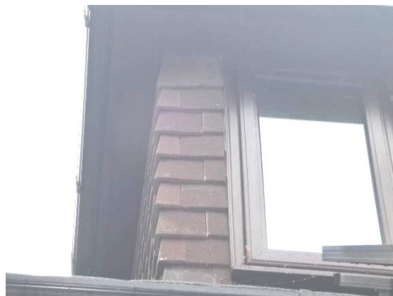
Photograph 12. Lifted hanging tiles (front elevation; TN4).
