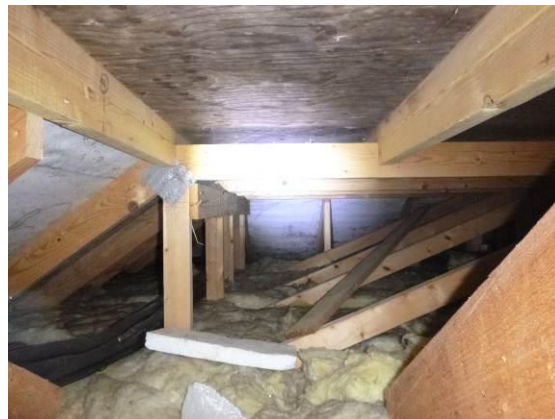
Photograph 23. Mansard dormer void with breathable/plastic roof lining.
