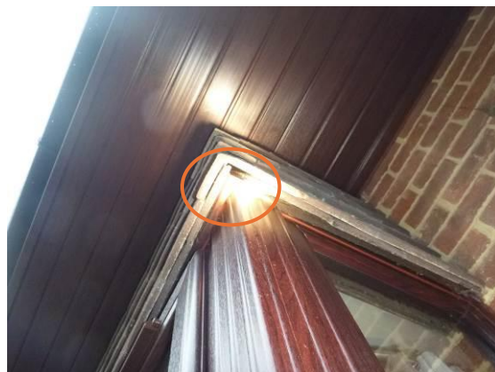
Photograph 15. Gaps behind front bay hanging tiles ( TN6 ).
