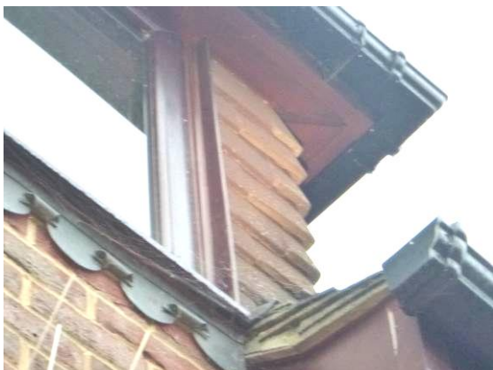
Photograph 11. Gaps under lifted hanging tiles (Rear elevation; TN4).
