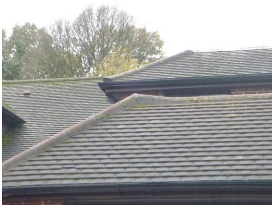
Photograph 3. Roof tiles mostly flat with intact ridge and hip tiles and mortar throughout (rear elevation).
