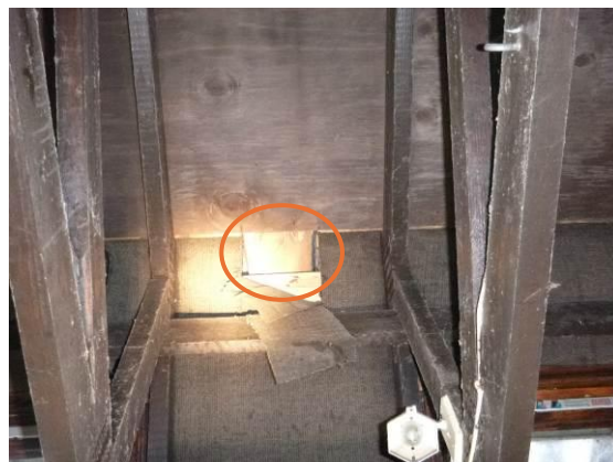
Photograph 10. Tear in underside of walkway felt (TN3).
