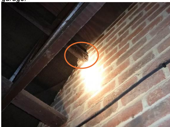
Photograph 9. Gap between timber and brickwork under walkway (TN3).
