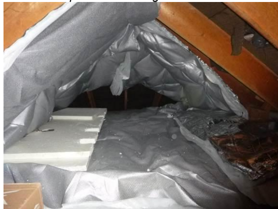
Photograph 25. Additional foil lined insulation covering the roof and floor at northern end of void (TN9).
