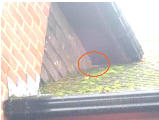
Photograph 13. Gap where dormer joins roof (rear elevation; TN5 ).
