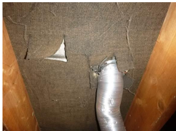
Photograph 21. Occasional tears around flues (TN7).
