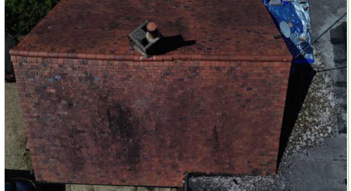
Main Dwelling roof arial view
