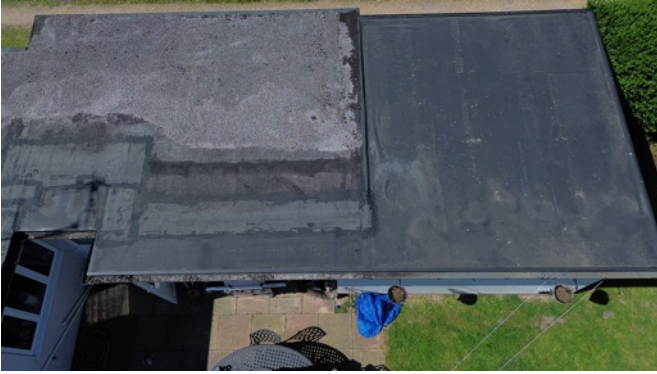
Flat roof arial view
