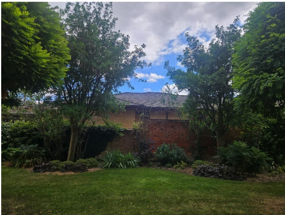
View from Remenham Row looking towards the existing north elevation of Thamesfield Retirement home.
